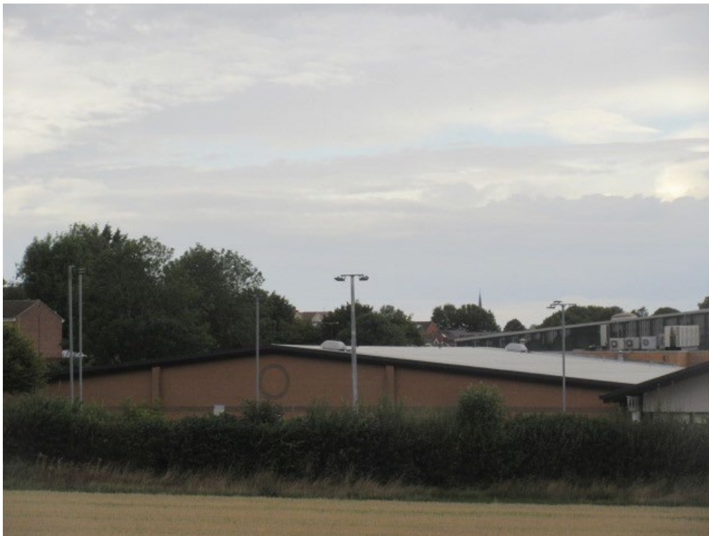
Plate 6: View from north west of site towards central Saffron Walden
