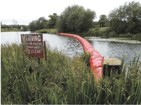
a A safety boom upstream of a weir should be installed at an oblique angle to direct debris towards one bank where it can be removed.
