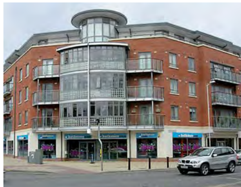
Image 87 Mixed-use building with active frontage
