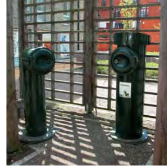
Image 79 Domestic waste chutes to underground storage, Malmö
