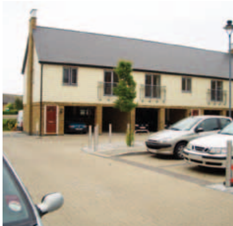
Undercroft parking facing onto central parking court
