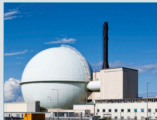
Dounreay Fast Reactor
