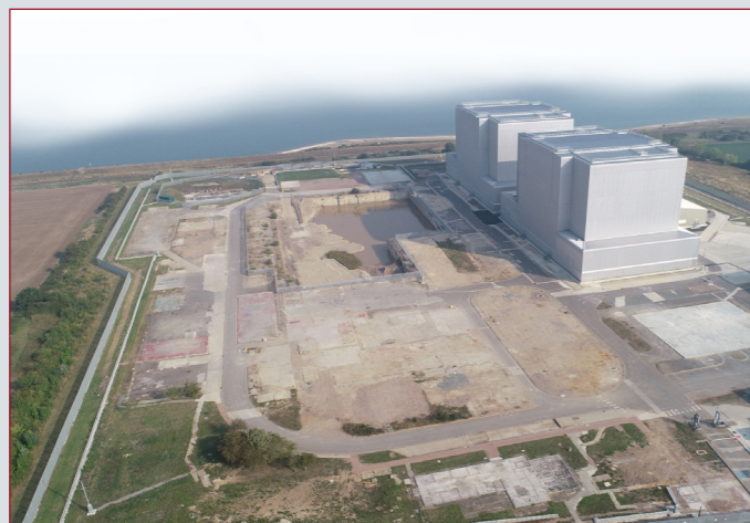
Bradwell in care and maintenance
