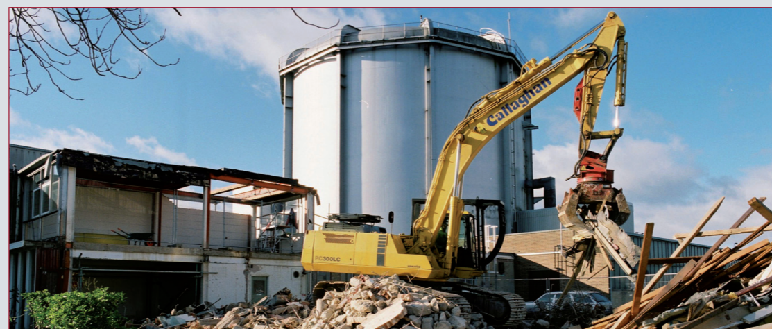
Demolition work at Harwell
