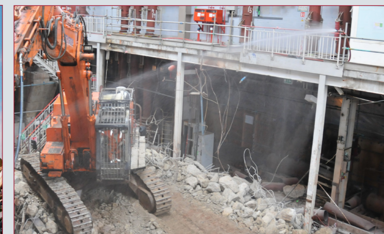
Turbine hall demolitions
