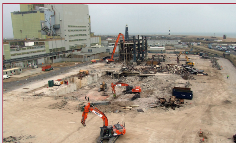
Demolition work at Dungeness
