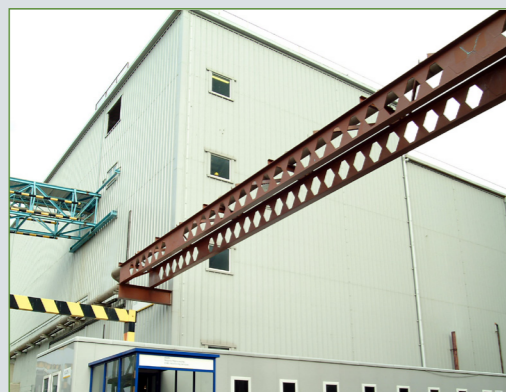
Magnox Reprocessing Plant
