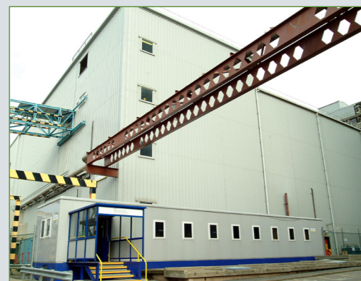
Magnox Reprocessing Plant
