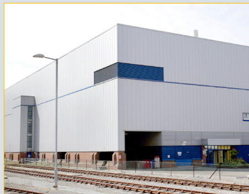
ILW Treatment and Storage at Sellafield
