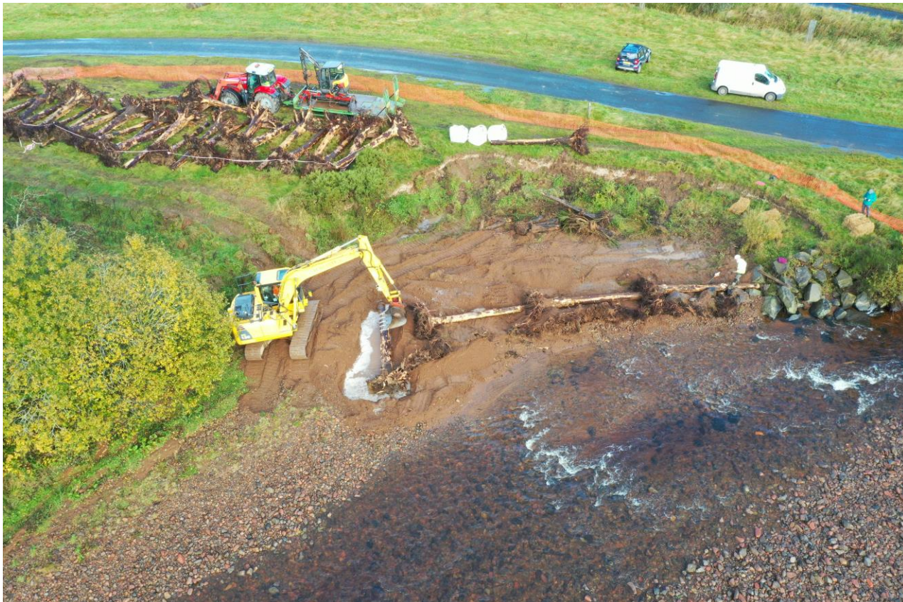
Figure 5: this picture shows the ‘root-wad’ technique used on the River Breamish to stabilise riverbanks and where the risk is more focused and localised.
