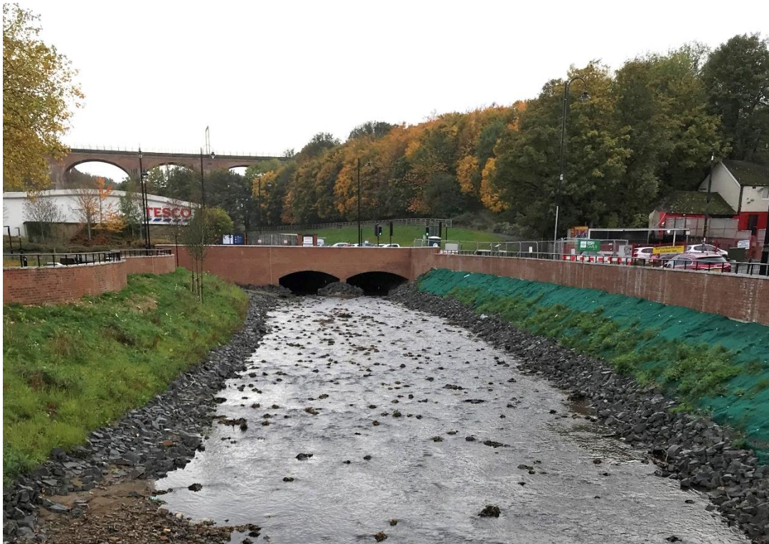
Figure 3: Chester-le-Street Scheme. Previously culverted, scheme has 'day lighted' the Chester Burn through Chester-le-Street.
