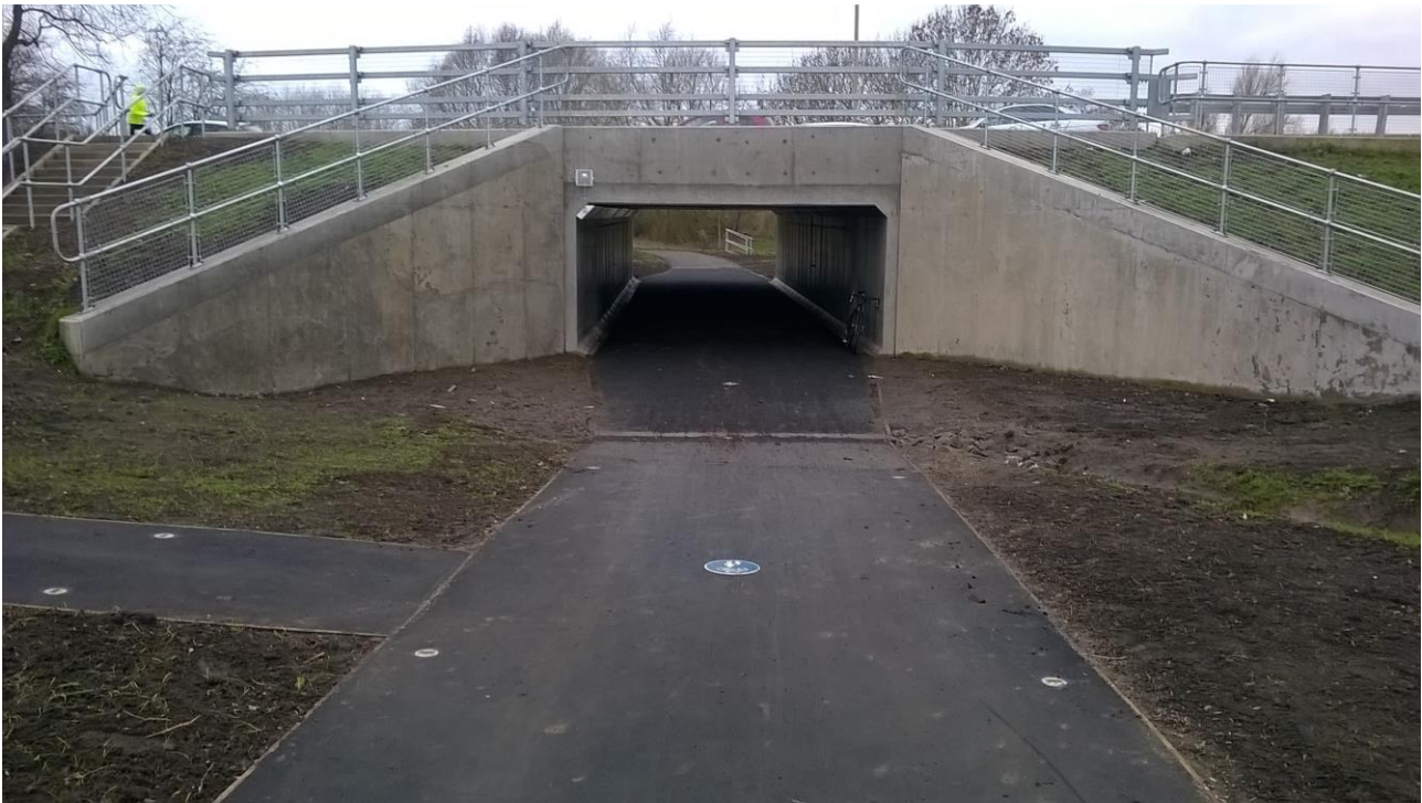
Figure 6: Loughborough Road flood relief culvert
