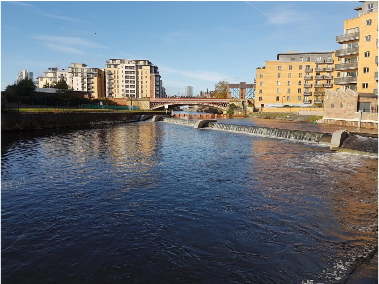
Figure 4: Leeds Flood Alleviation Scheme 1
