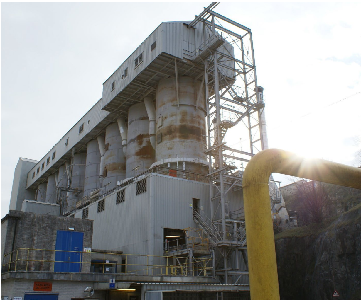
Figure 11: Tarmac Buxton Lime shaft kilns and kiln building
