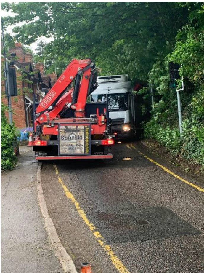
Road blocked at traffic signals (Grove Hill)
