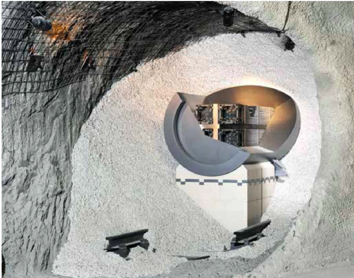
Figure A2-2: Cutaway model of the Nagra ITA concept for SF [A2.3].
