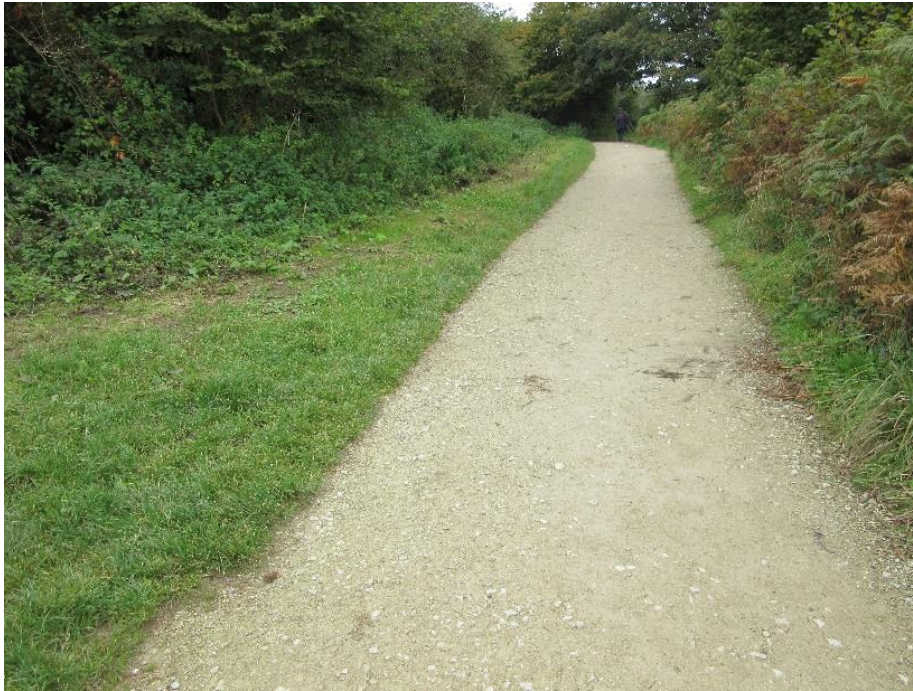
Photo 7. Route Section LCH-4-S011 BW – compacted gravel – good condition (29 Sept 2017)
