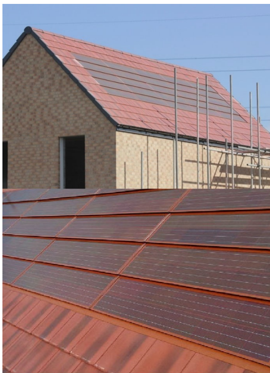
Integrated photovoltaic clay-type roof tile (source: Romag)
