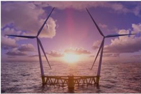
Twin Turbine Floating Foundation
