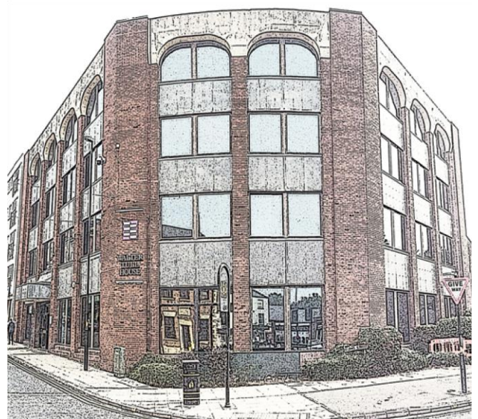
Bridge Street, Northampton Probation Service
