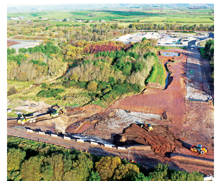
Progress being made on the haul road, in November 2021
