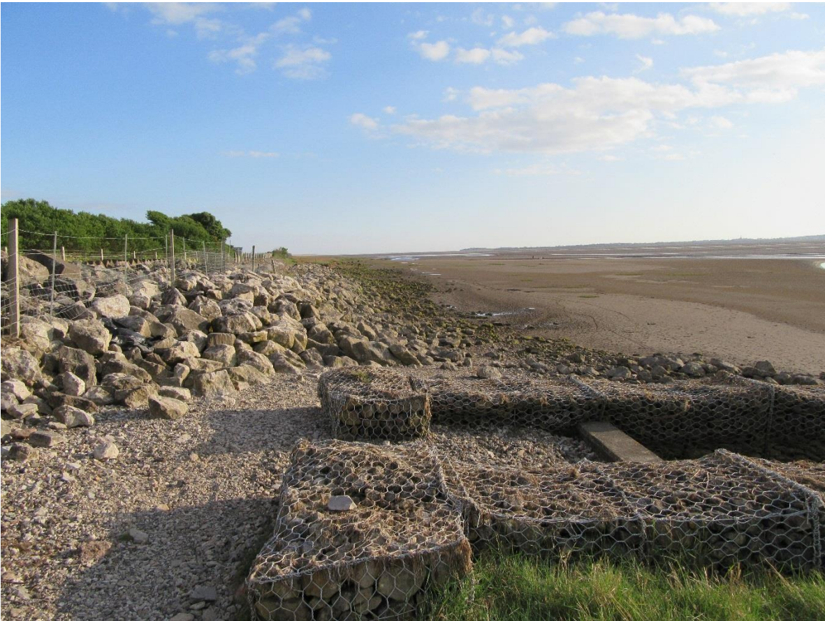
3. Rotten footbridge next to Kirkby Station that needs work on it.
