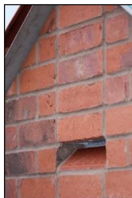
Figure 1: Habibat Bat Box faced with red brick, incorporated within wall at gable end.
