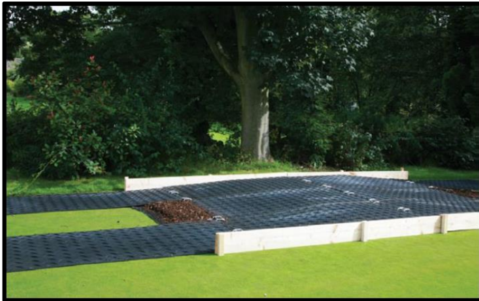
Figure 6 Examples of proprietary ground protection panels
