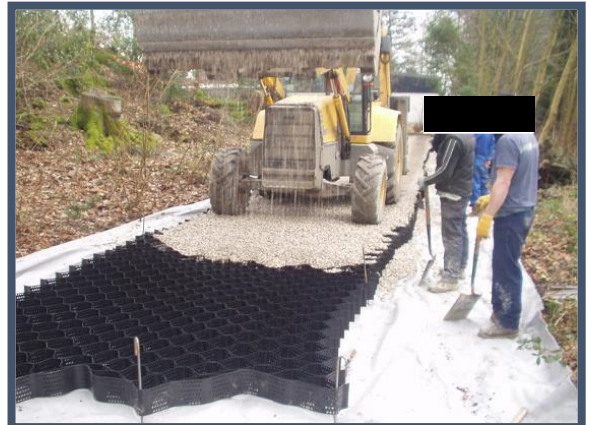
Figure 11 Examples of Cellweb filling with angular stone
