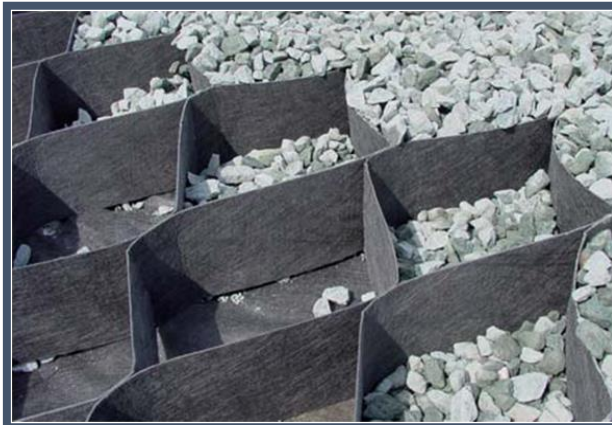
Figure 11 Examples of Cellweb filling with angular stone
