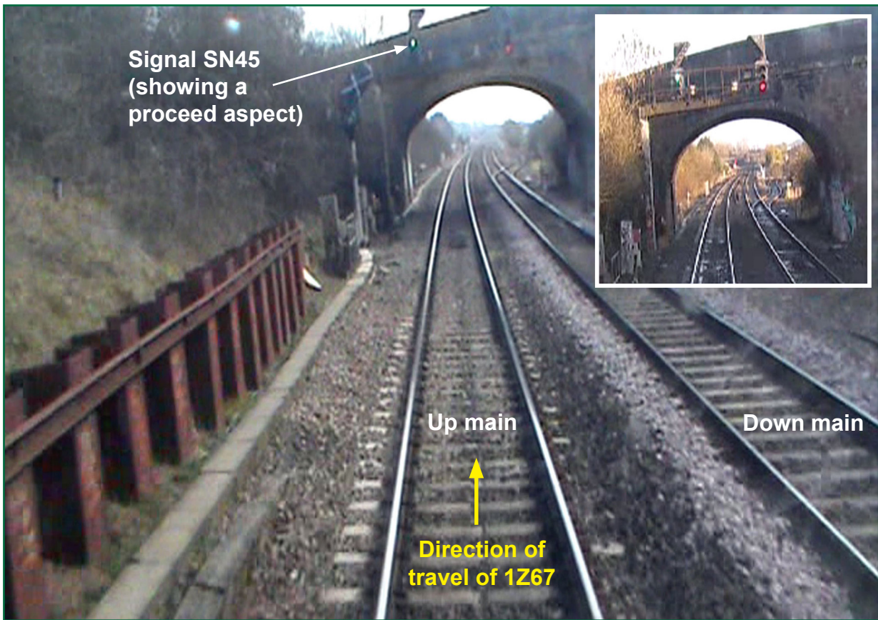
Figure 3: A video image of signal SN45 taken shortly after the incident. Inset figure shows an HD video image of the signal head taken in 2012 (images courtesy of Network Rail).
