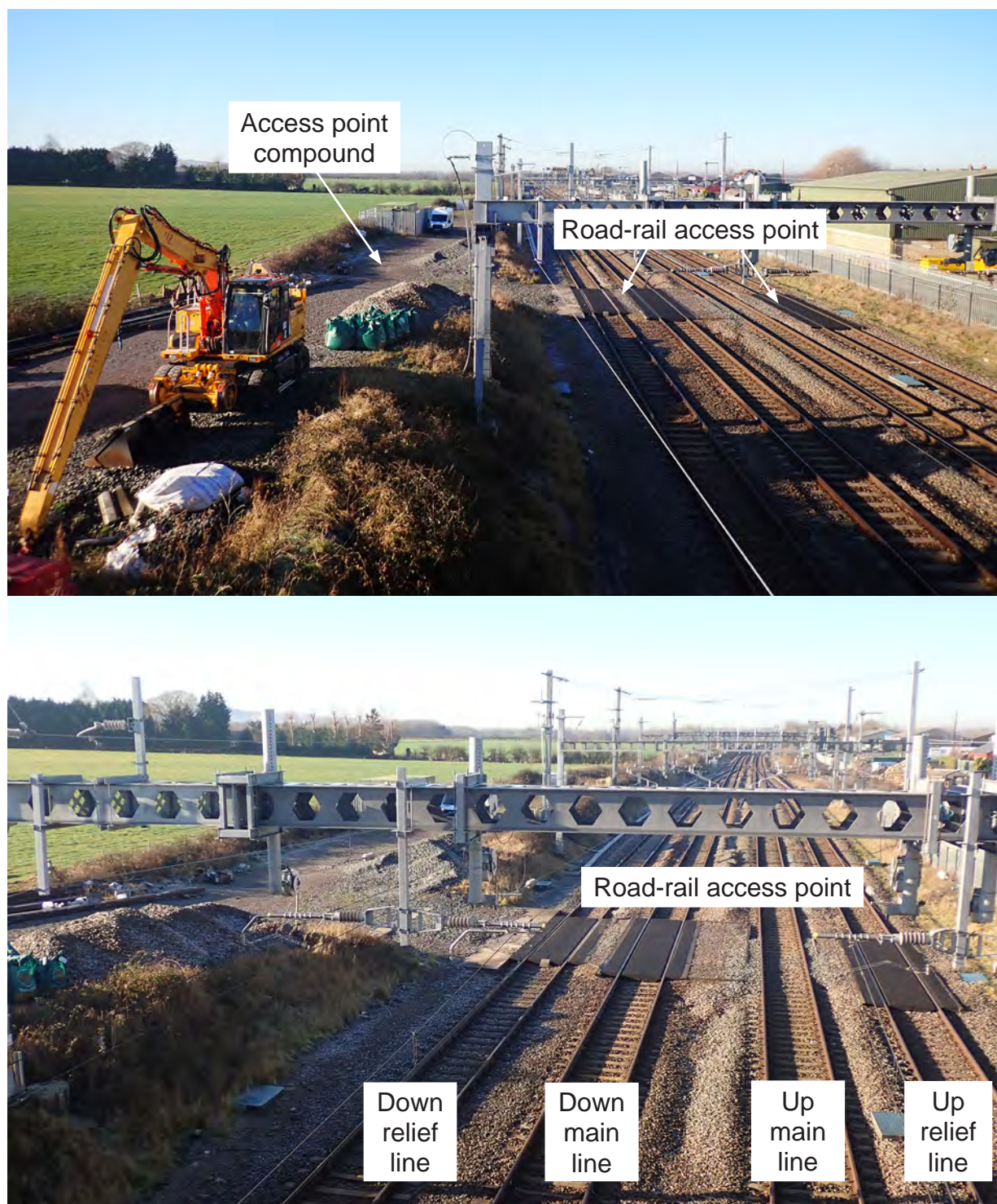
Figure 5: The road-rail access point at Challow
