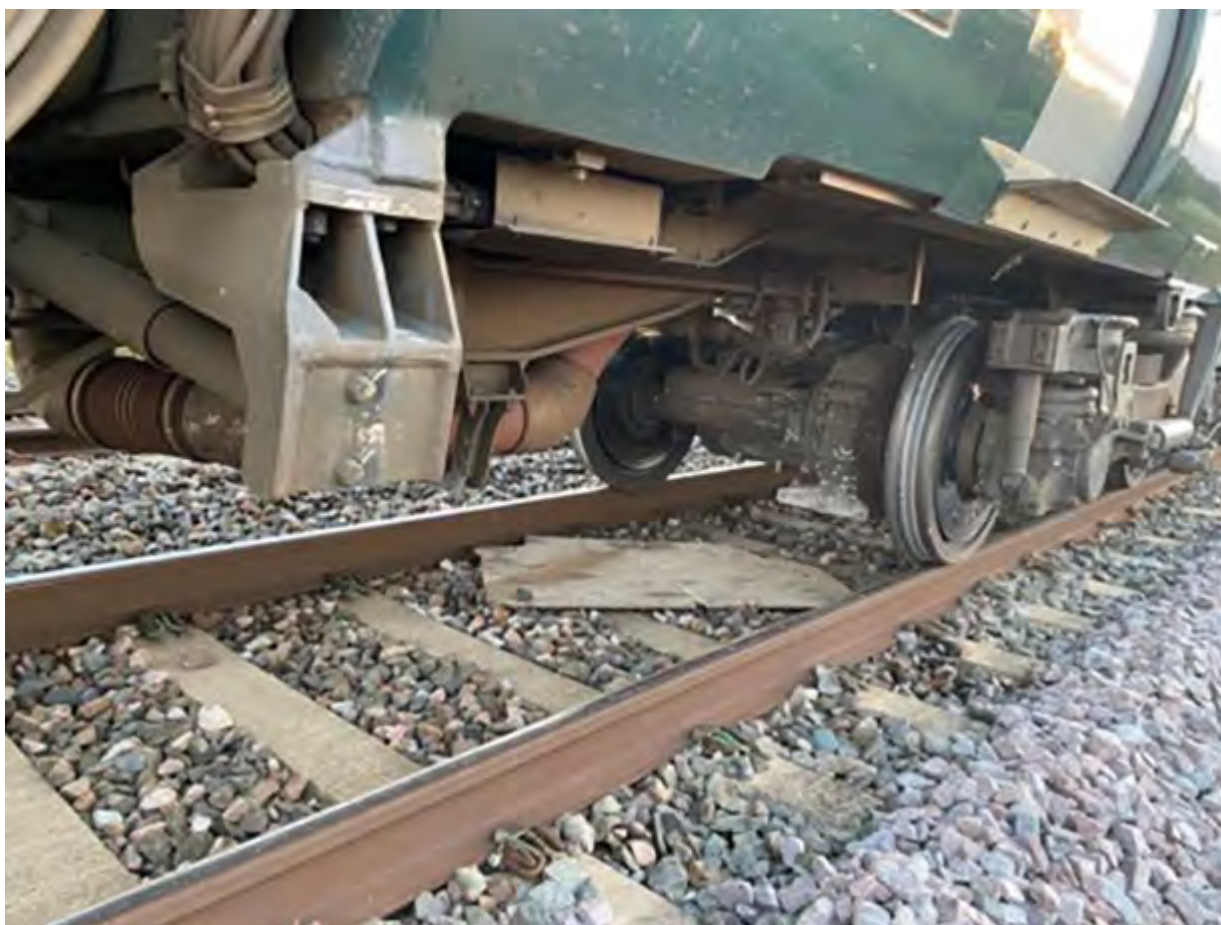
Figure 9: The hand trolley's wooden deck underneath the second vehicle (courtesy of Network Rail).
