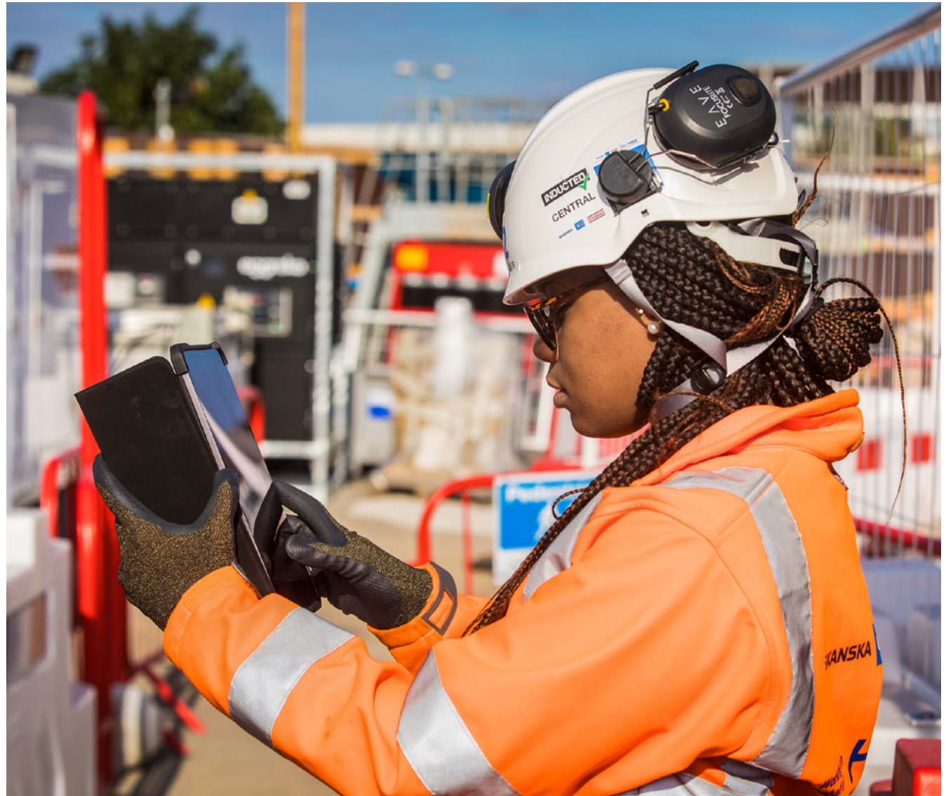
Engineer at the Westgate vent shaft in Ealing.
