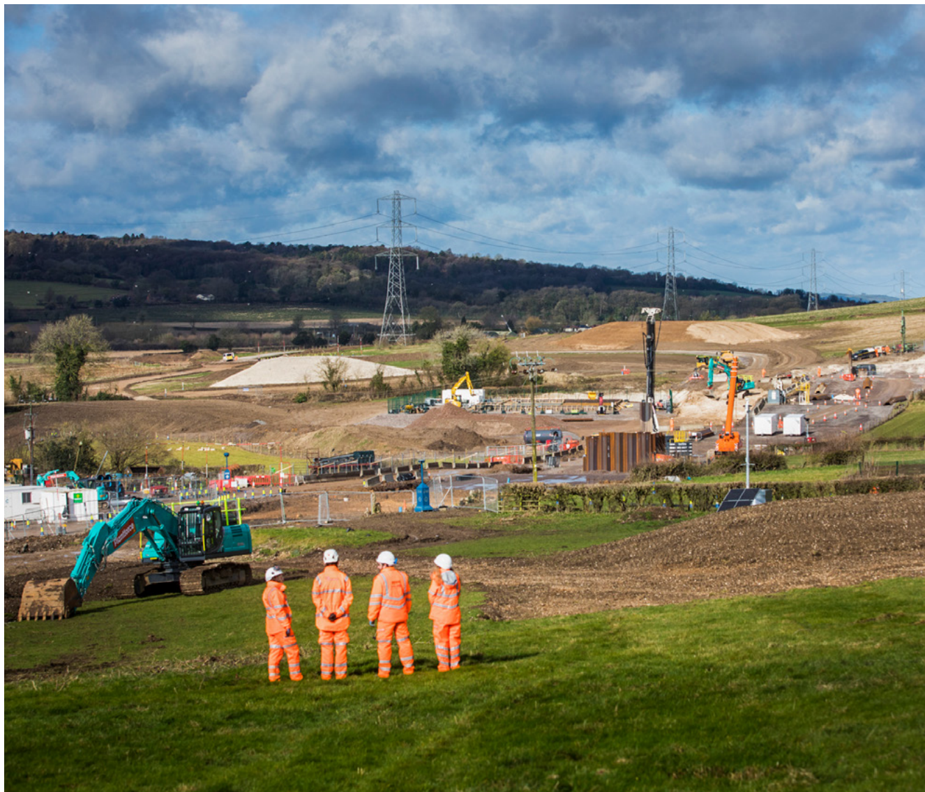
EKFB workers at Wendover Dean viaduct, Buckinghamshire.
