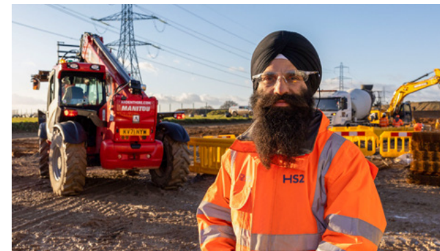
An HS2 worker at the north portal site in Buckinghamshire.
