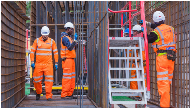
Workers fixing steel reinforcement for a propping beam.
