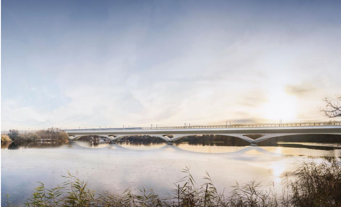
Colne Valley Viaduct
