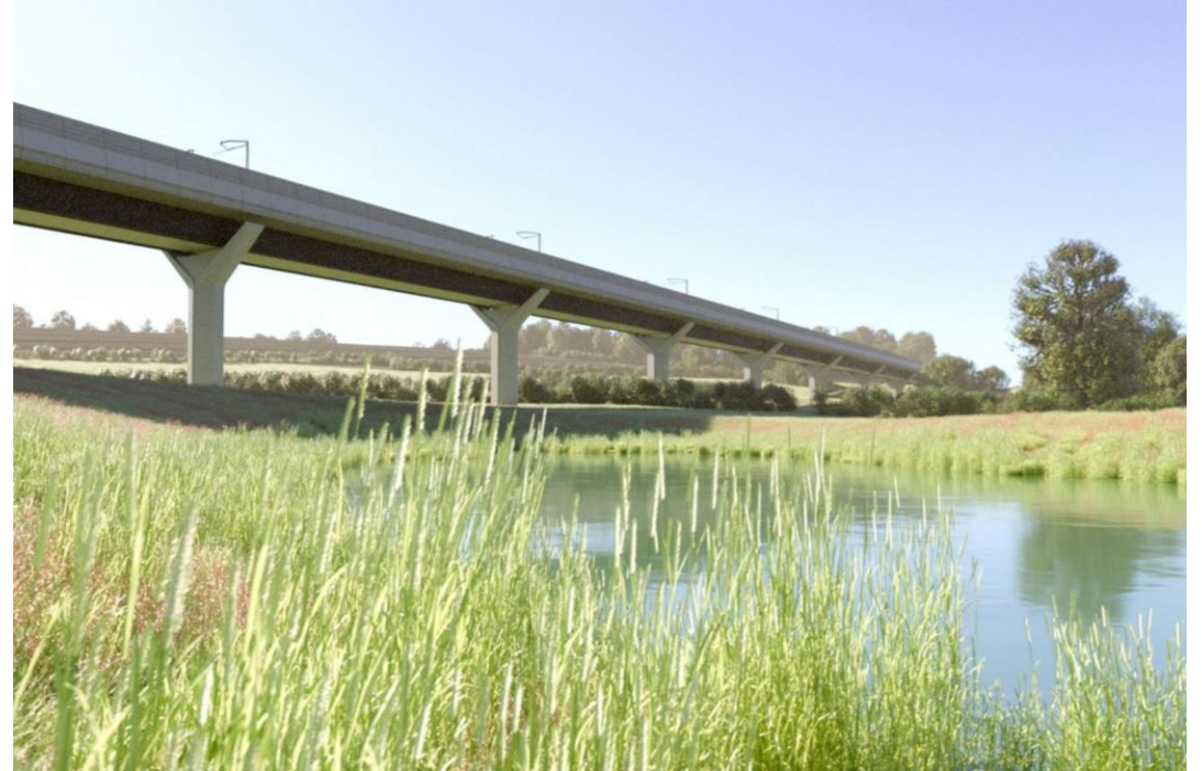
Wendover Dean Viaduct
