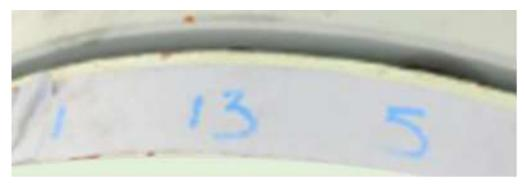
Note. The correct numbering of bolts should result in the odd-numbered bolts being around one side of the flange and the even-numbered bolts being around the other side.
