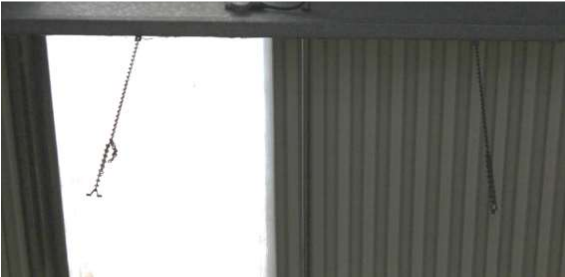
Photograph A. Suspension chains and 3 no. clips
