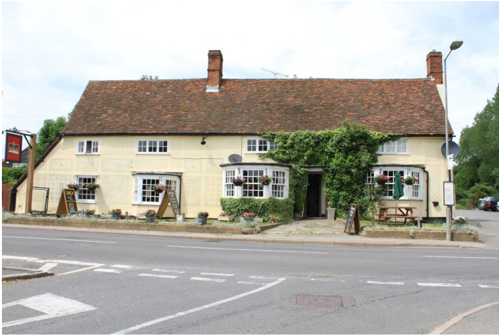
THE CROWN INN List Entry Number: 1305698 Grade II GV C18 timber-framed and plastered building. Two storeys Listing NGR: TL5382226342
