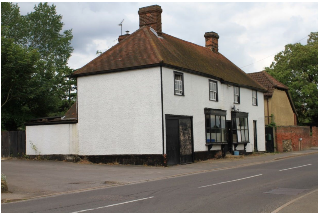
THE STORES AND HOUSE Name: THE STORES AND HOUSE List Entry Number: 1322535 Grade: II Late C18 or early C19 timber-framed and plastered building. Two storeys. (Formerly Village Stores)
