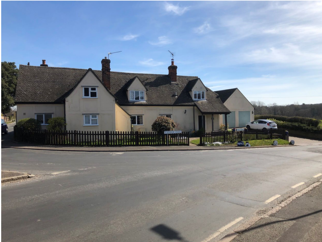
1 and 2 The Cross List Entry Number: 1322511 Grade II Early C18 timber-framed and plastered cottages on a T shaped plan. Listing NGR: TL5384226325
