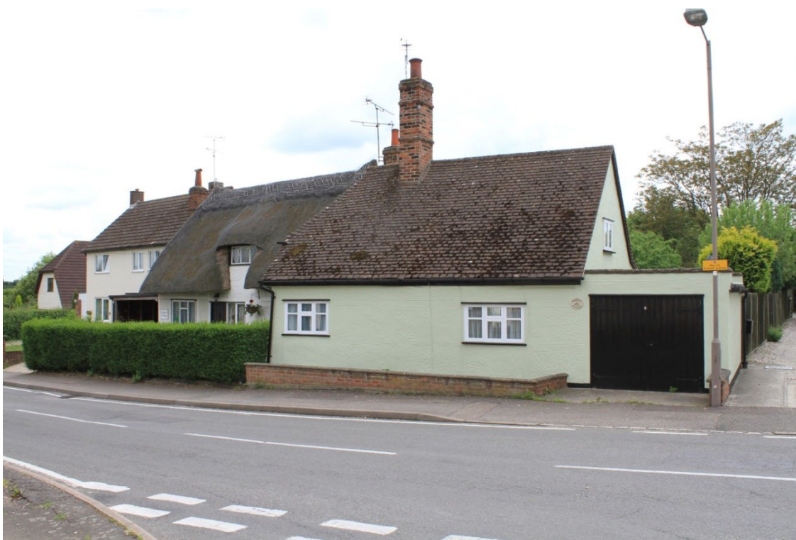
Elsenham Cross No.5 Sophie's Cottage List Entry Number: 1112368 Grade II GV Small timber-framed and plastered house with late C18 or early C19 external features Listing NGR: TL5382826306
