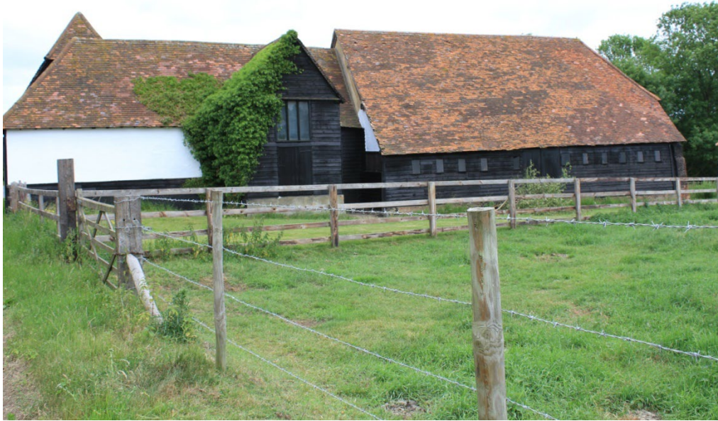
BARNS TO WEST OF ELSENHAM PLACE FRONTING ROAD Grade: II Listing NGR: TL5401626405 An L-shaped range of C17 and C18 timber-framed and weather-boarded barns, with some plaster on the west side. Roofs tiled. A large C17 barn extends to the east and west with a half hipped roof and C18 barns extends to the south at the west end. List Entry Number: 1171188
