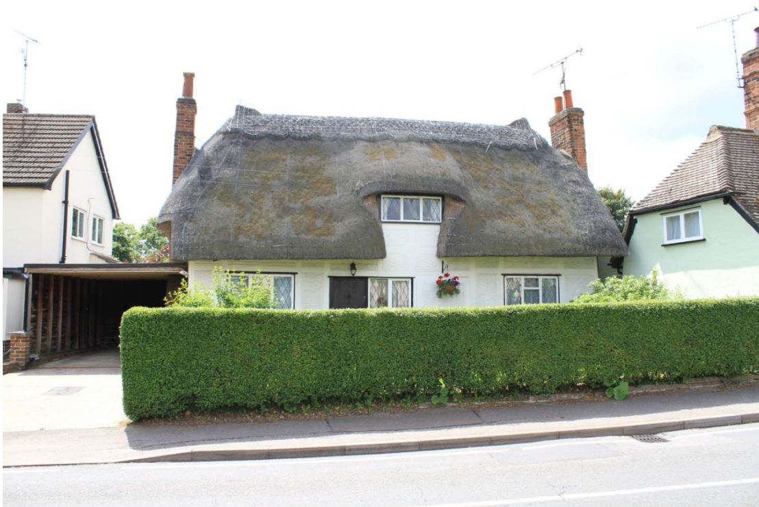
ELSENHAM THE CROSS TINKERS COTTAGE List Entry Number: 1305747 Grade: II Small C17-C18 timber-framed and plastered building
