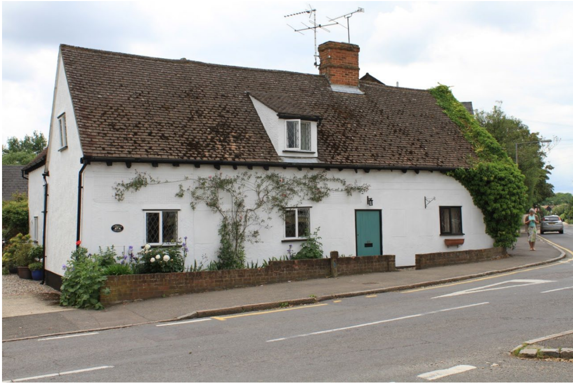
VILLAGE HALL COTTAGE Now Known as Camelia Cottage List Entry Number: 1305746 Grade: II Early C18 timber-framed and plastered house. One storey and attics.
