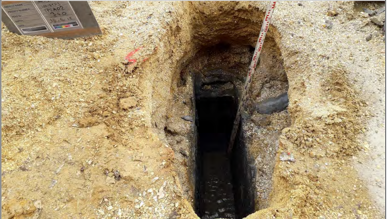
TP2A02 Trial Pit. Depth 3.40m
