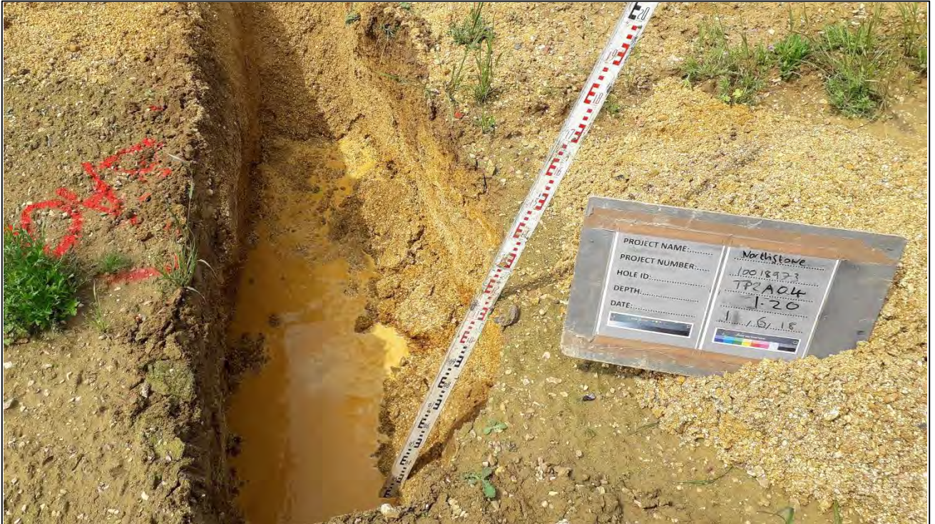
TP2A04 Trial Pit. Depth 1.20m
