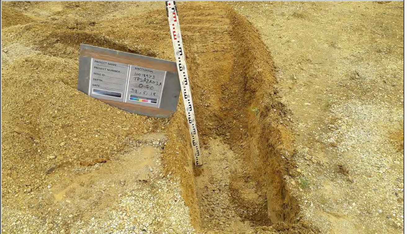
TPSA2A03A Trial Pit. Depth 0.50m
