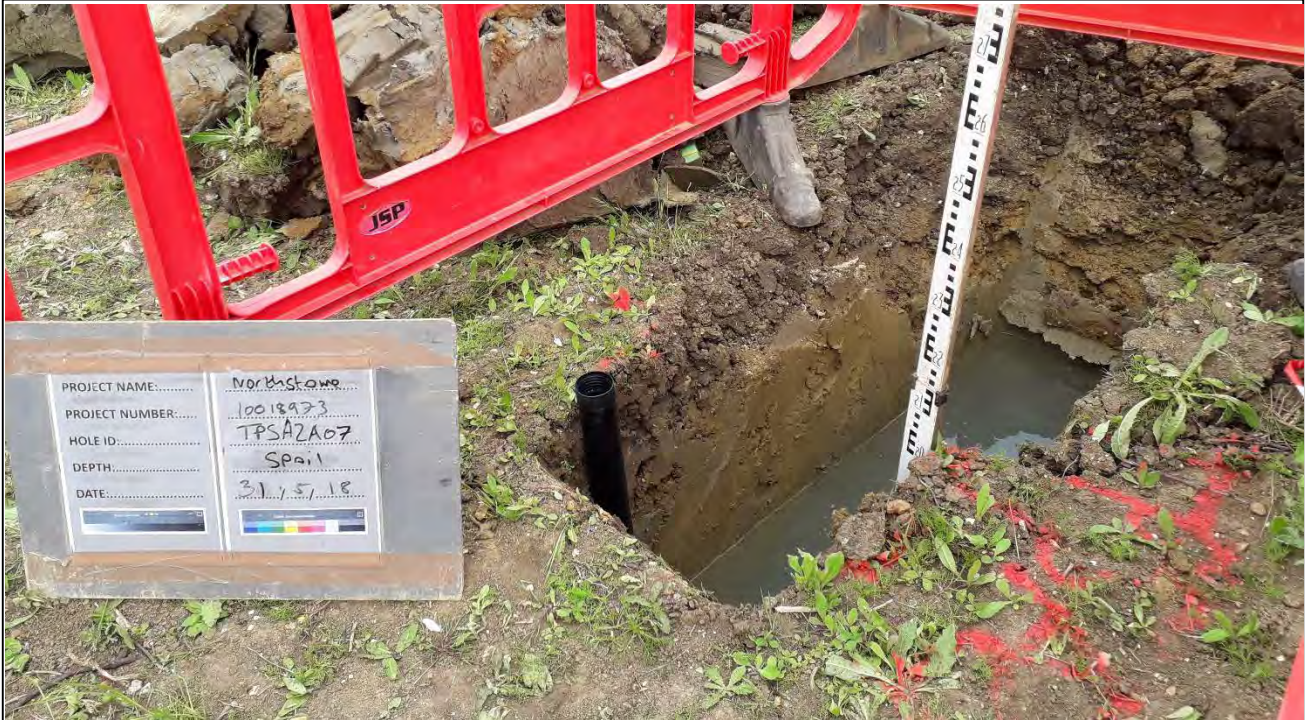
TPSA2A07 Trial Pit. Depth: 2.10m
