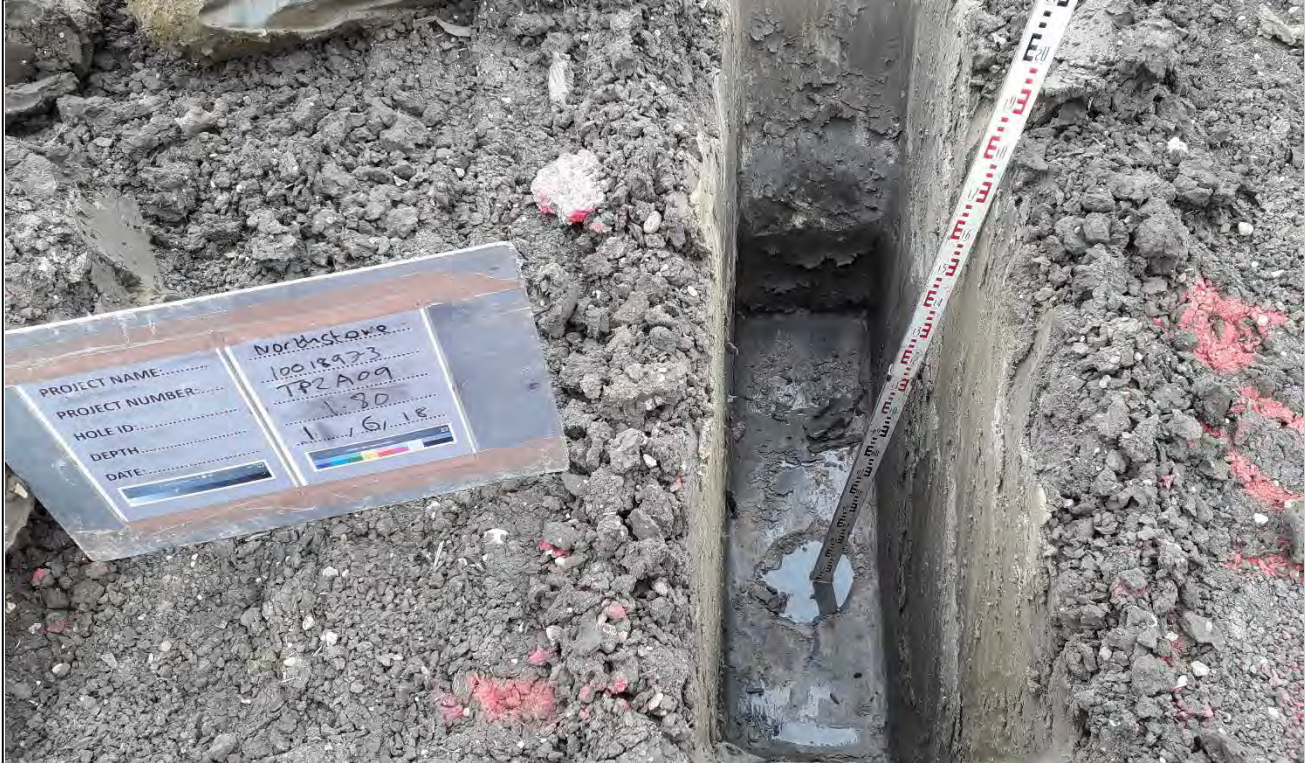
TP2A09 Trial Pit. Depth 1.80m
