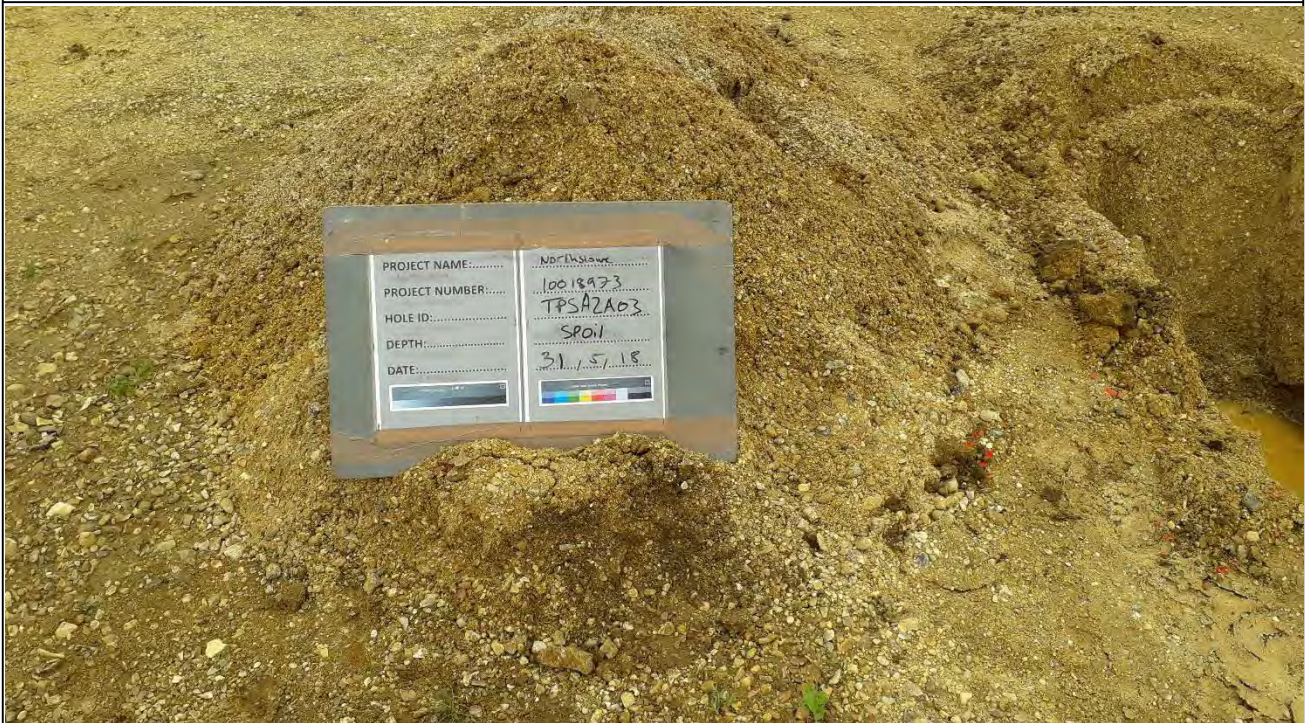
TPSA2A03 Trial Pit Spoil
