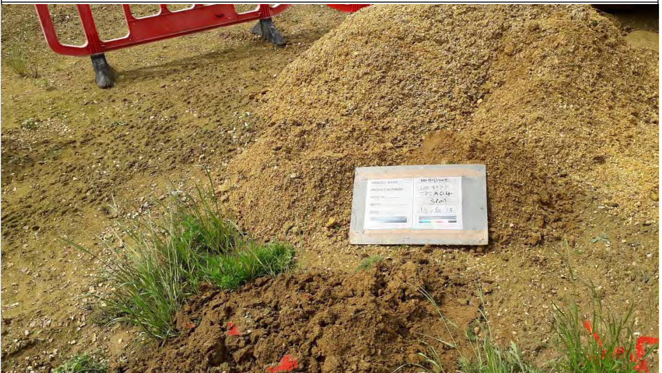
TP2A04 Trial Pit Spoil
