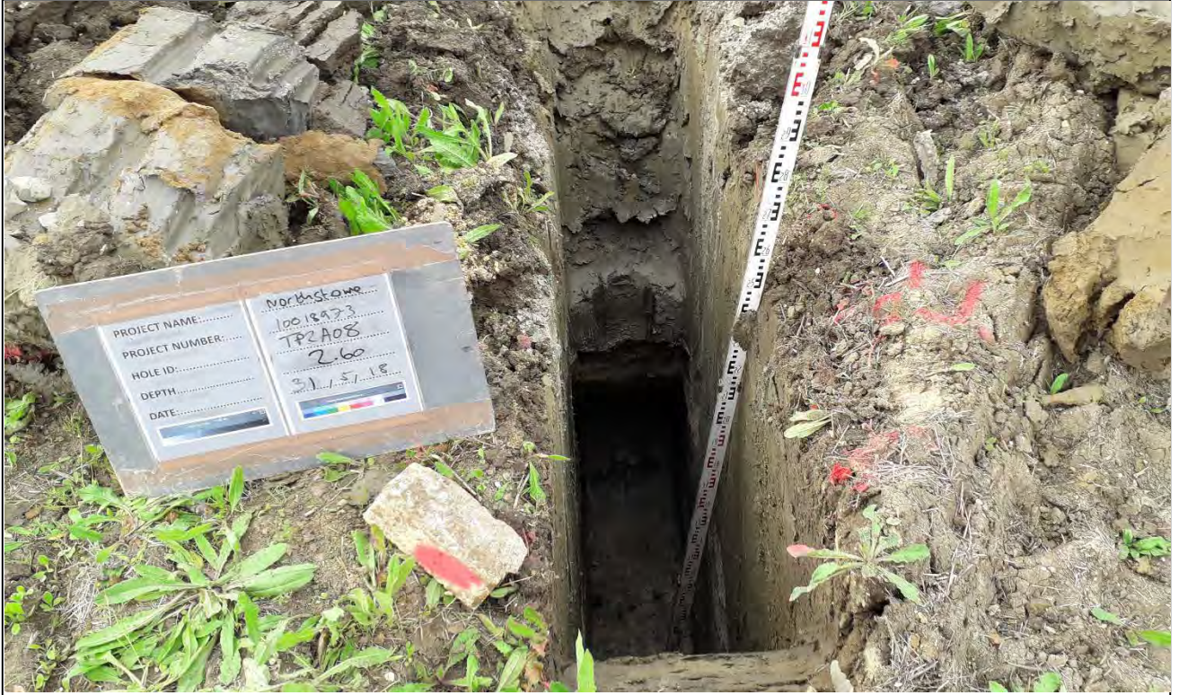
TP2A08 Trial Pit. Depth 2.60m
