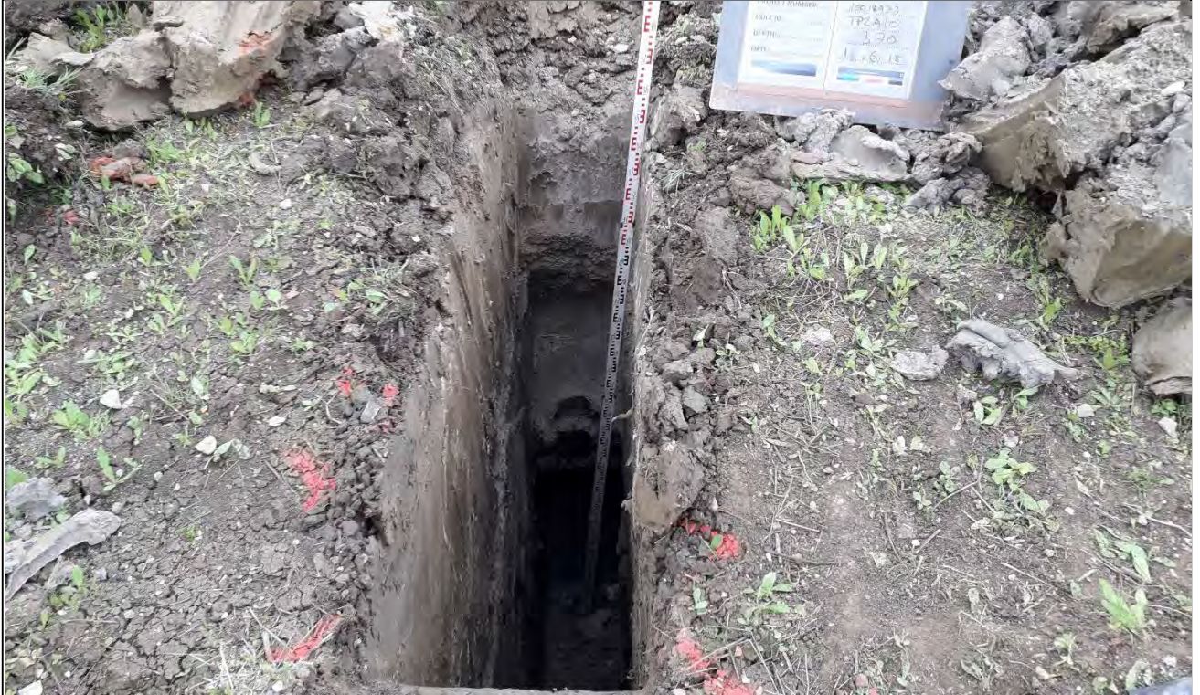
TP2A10 Trial Pit. Depth 3.60m
