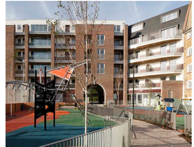
Estate regeneration including new mixed tenure homes, a community centre and a Multi-Use Games Area for social and physical well-being. Bourne Estate, Holborn, London.
