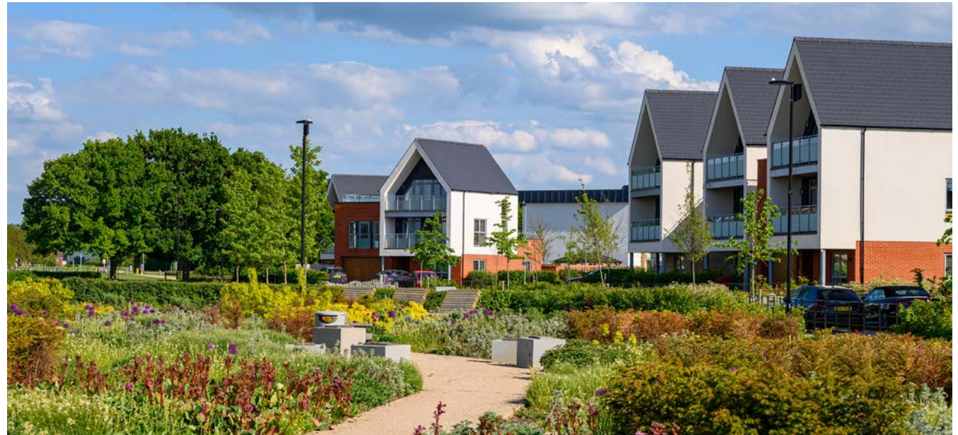
High quality green public spaces provide key pedestrian links to local facilities, a range of outdoor amenity including play areas, and a net gain in biodiversity. Beaulieu Park, Chelmsford.
