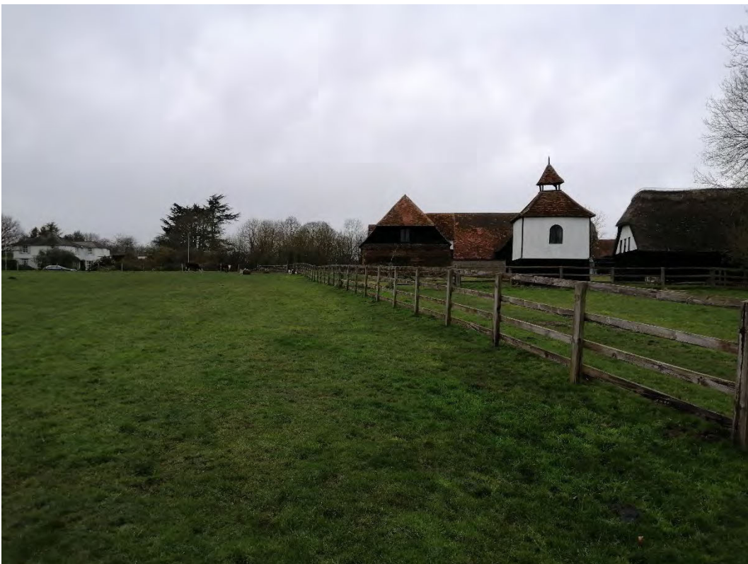
Photo 4: Looking north along northeastern boundary, note Elsenham Place beyond the boundary.
