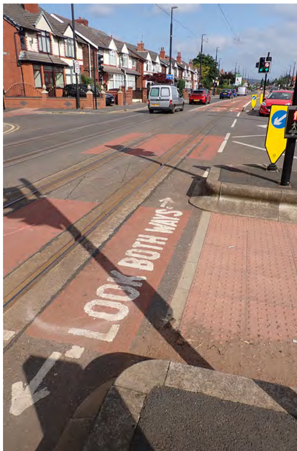
Figure 15: 'Look Both Ways' markings painted onto the road surface
