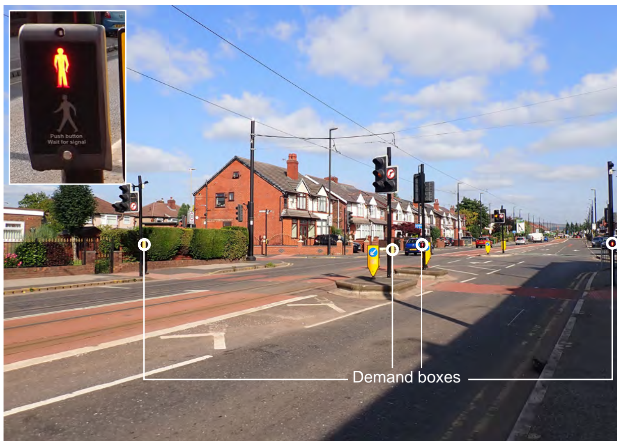
Figure 4: general view of the Puffin crossing across Droylsden Road (looking east), with (inset) demand box showing 'red standing man' indication
