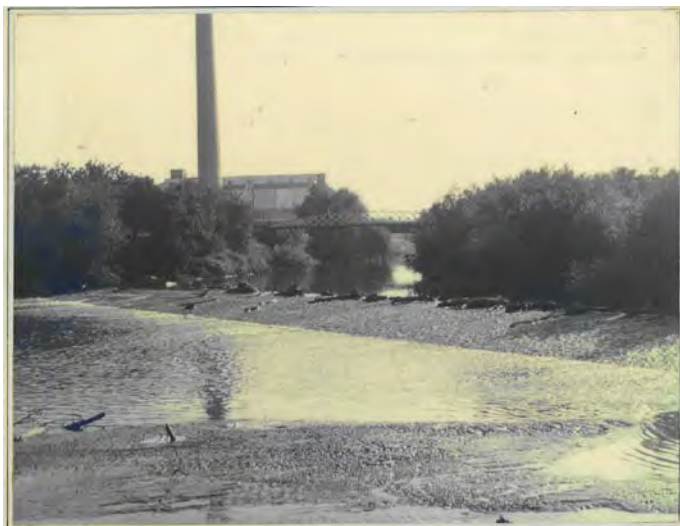
RIVER SEVERN. – LLANTHONY WEIR and EAST CHANNEL. 20th AUGUST 1976.
