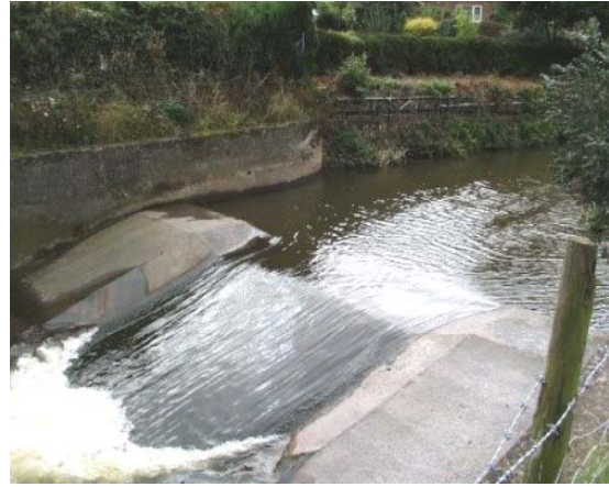
2. V Shaped broad crested weir
