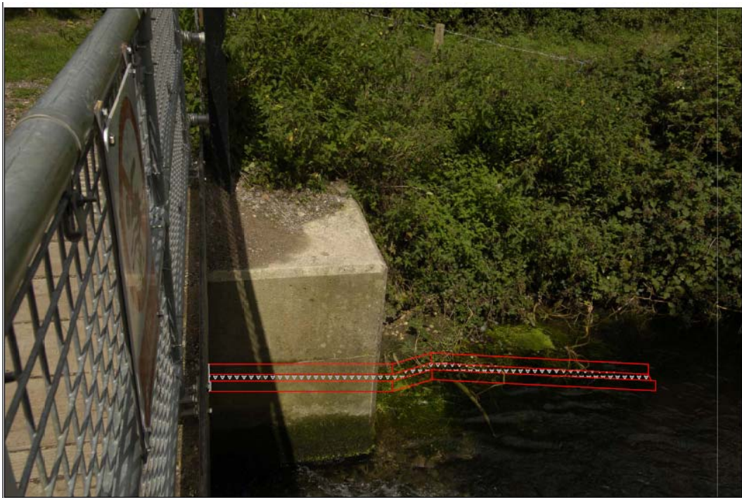
Figure 8.2: The position of the pass entrance. Note that the pass will be cranked towards the bank. This is to maximise the opportunity for eels to find the flow coming down the pass –eels migrating upstream routinely stay close to the banks.
