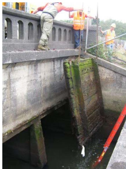
Figure 6.2 shows a large wooden flap being removed from a site in Washington State, US. It is clear that in this condition the seal would have been far from perfect – even though the gate was still effective at minimising back-flow when closed.
