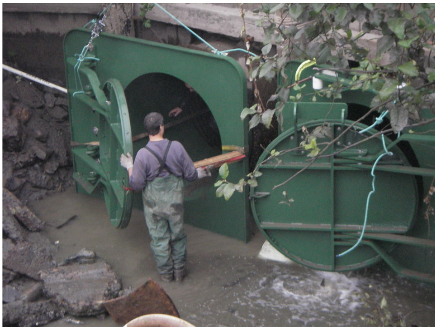
Figure 6.13: Side-hinged gates are fitted to replace top-hung flaps at Schneider Creek, Washington State, US.
