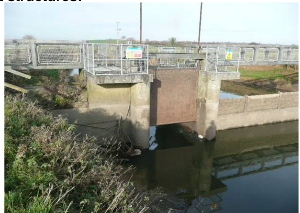
B. Large penstock sluice
