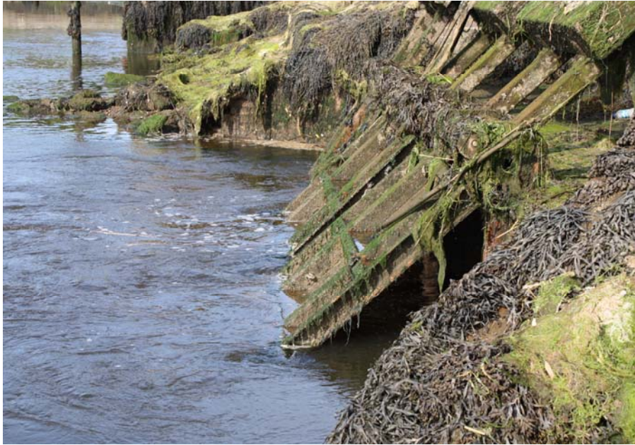
Figure 7.23: Counter-weighted tidal flaps on the River Lymington, Hampshire. These tend to open further and remain open longer than conventional flaps of similar weight.
