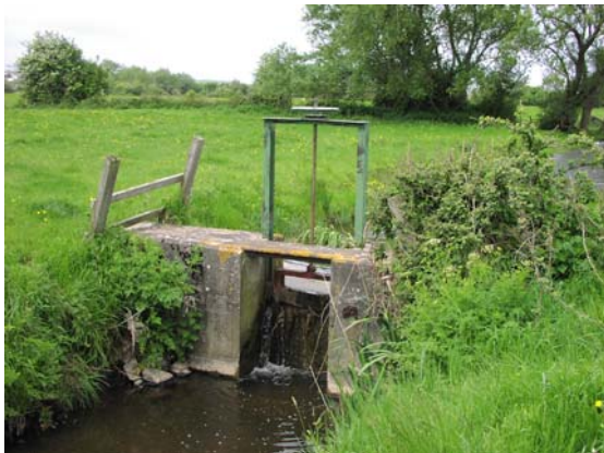
C. Small penstock sluice
