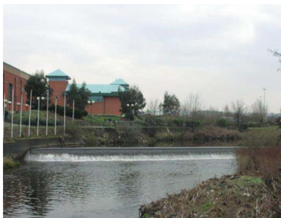
Figure 4.4 Rectangular Weir
