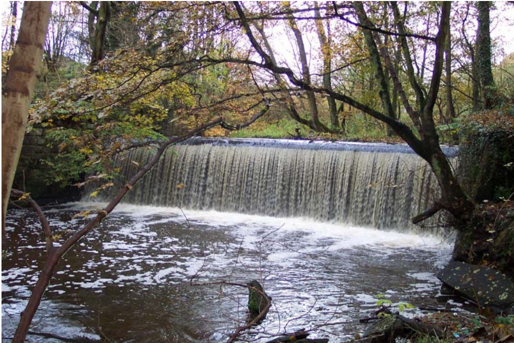
Figure 1: Duxbury Weir is an obstruction on the River Yarrow. (Note: There is now a fish pass at this site to make it easier for fish to travel upstream).
