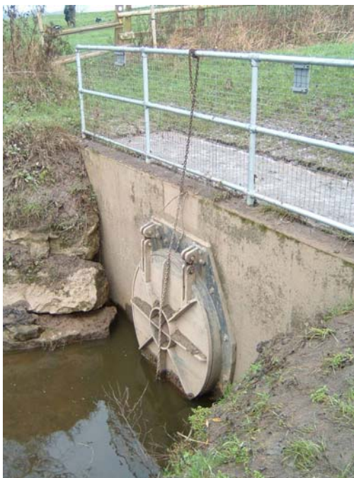
Figure 6.4: Round top hinged tidal flap gate
