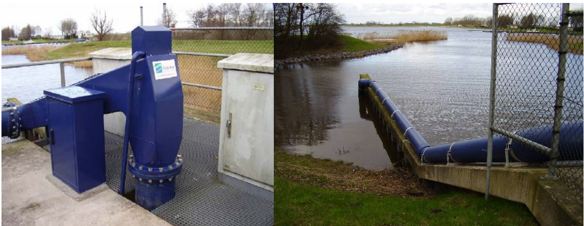
Figures 7.29 and 7.30: Eel-only fish siphon. Pipe encloses eel brushes only. This siphon was installed on the River Roggebotsluis near Kampen in February 2007. The ladder enables migration of eels between Lake IJsselmeer and Lake Veluwe.
