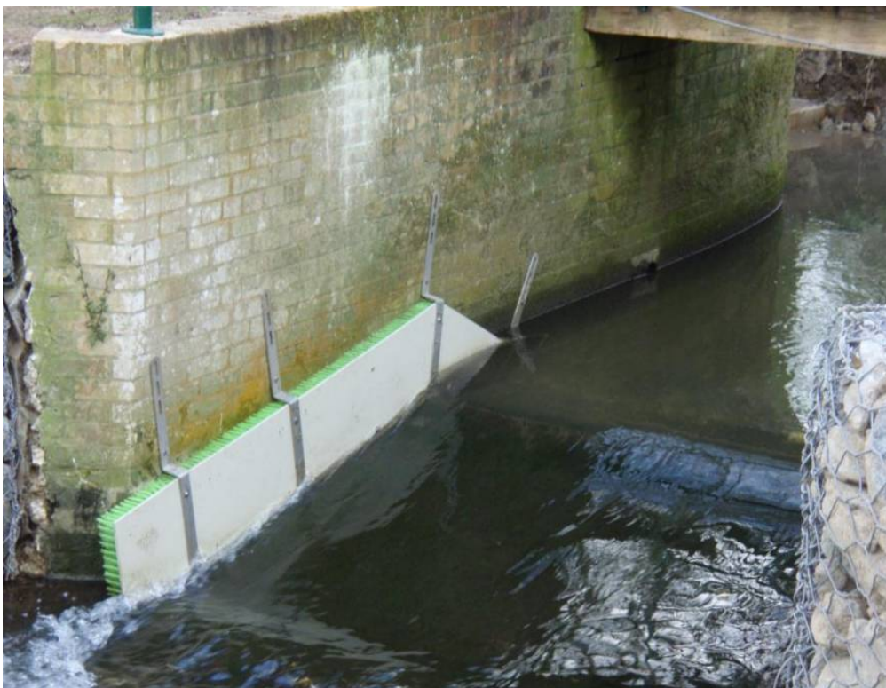
Figure 4.13: Installed pass, showing brackets and fixings
