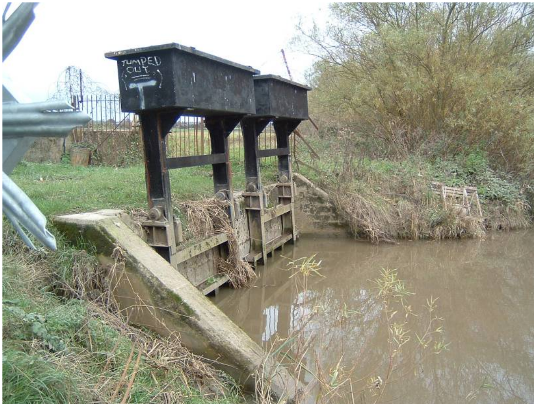
Figure 7.25: Counter-balanced gates on the River Leadon, Gloucestershire. Note that the gates are shut because of tidal influence. They soon open wide with the ebbing tide.
