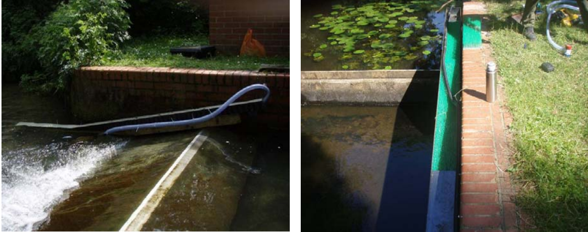
Figures 4.15 and 4.16: Crawling gutter of fabricated steel with bristle medium installed and lower lids fitted.
