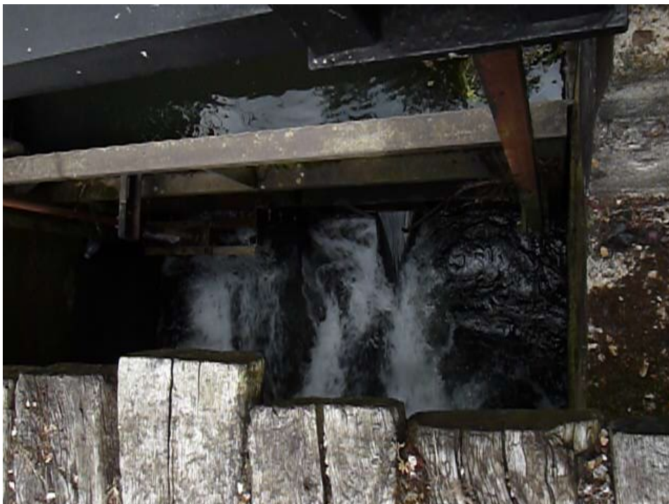
Figure 7.18: Mouse hole on sluices on the River Test. As the downstream water levels rise, fish can pass through hole.
