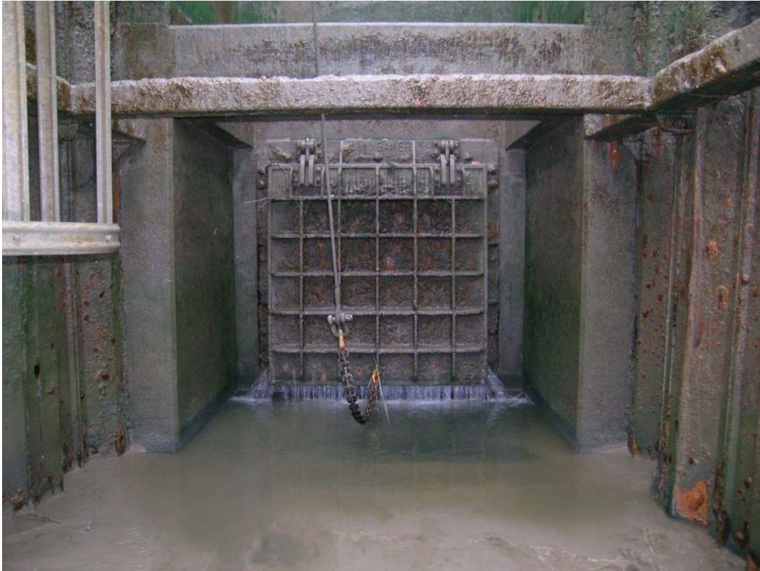
Figure 6.15: Two metre square section tidal flap at Havering, Essex. This drains an area of Havering Marshes to the Thames Estuary.
