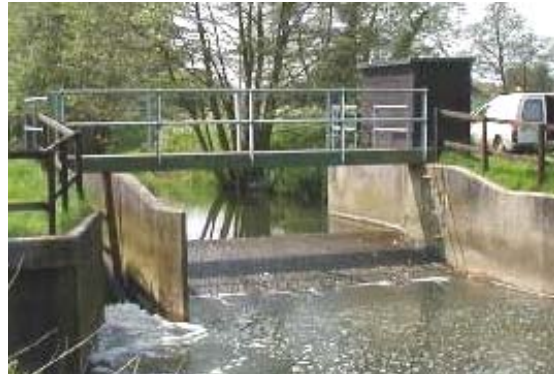
Figure 4.3 Compound Crump weir
