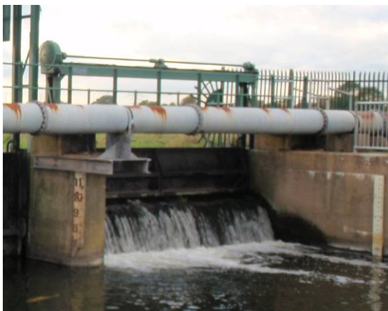
C. Small penstock sluice
