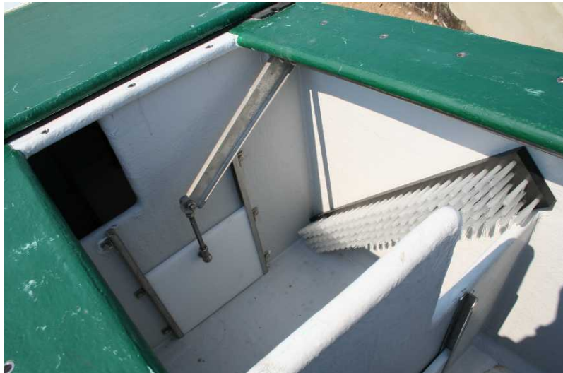
Figure 7.32: The top of the fish ladder. Note the eel brushes which aid eel migration.
