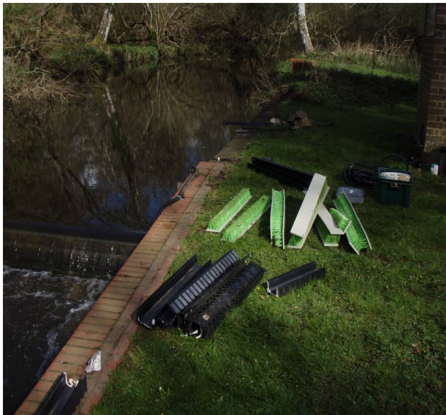
Figure 4.19: Gutter pass materials and bristle mat substrate being assembled on site.
