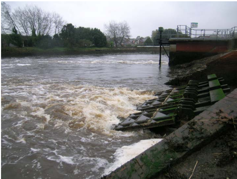
Figure 7.24: Counter-weighted tidal flaps on the River Lymington. Shown fully open during a spate.
