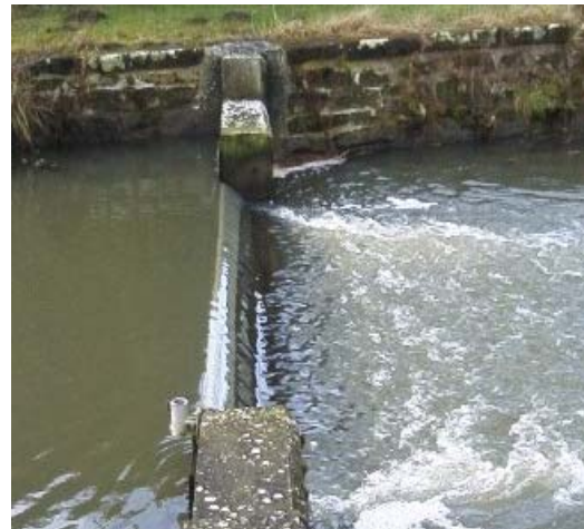
4. Contracted thin plate weir
