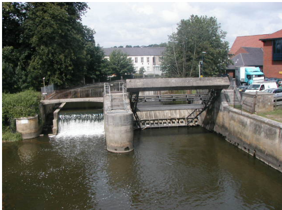
A. Radial gate, right.
