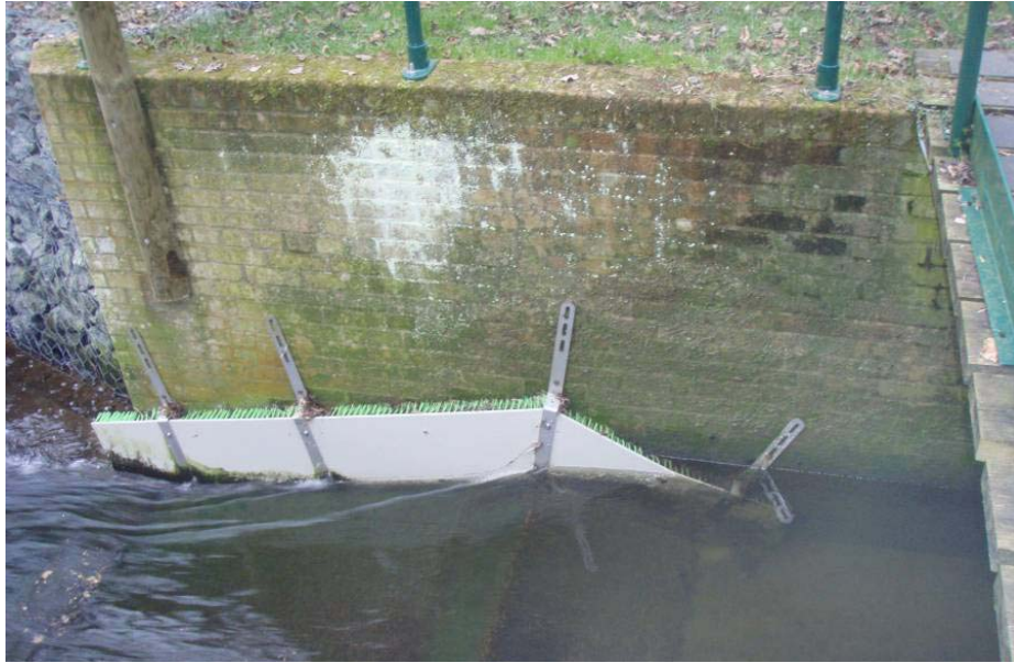
Figure 4.1: Crest section of installed pass
