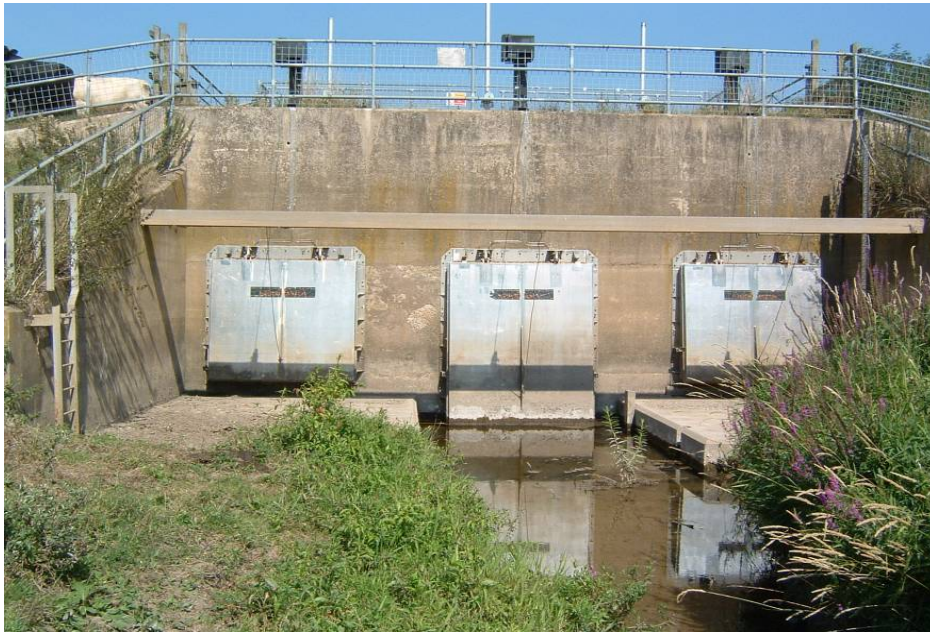
Figure 6.5: Square, top-hinged tidal flap gate
