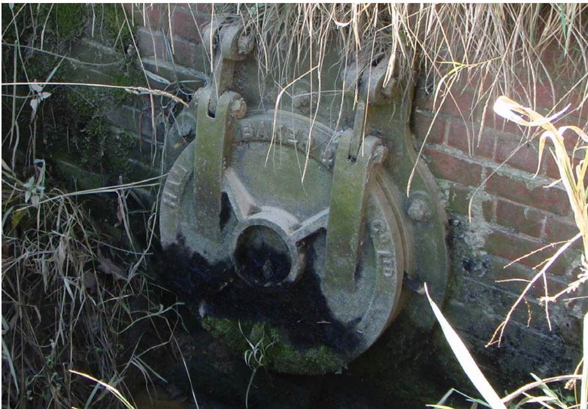
Figure 6.14: A pegged tidal flap: a piece of wood at the 3 o'clock position holds the flap ajar.
