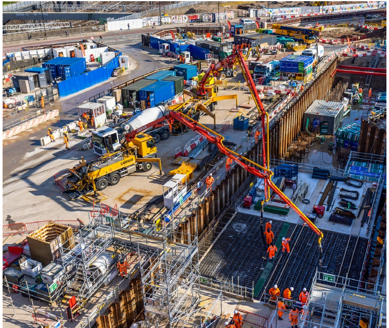
The Euston throat site on the approaches to the new station.
