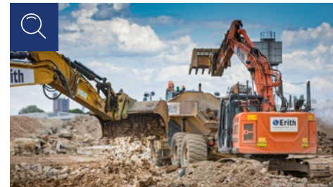
Demolition materials are being reused.
