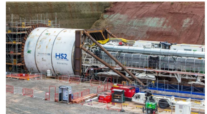
Dorothy, the tunnel boring machine at Long Itchington Wood.
