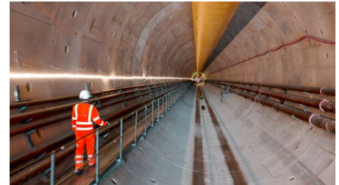
Progress on the Chiltern tunnel.
