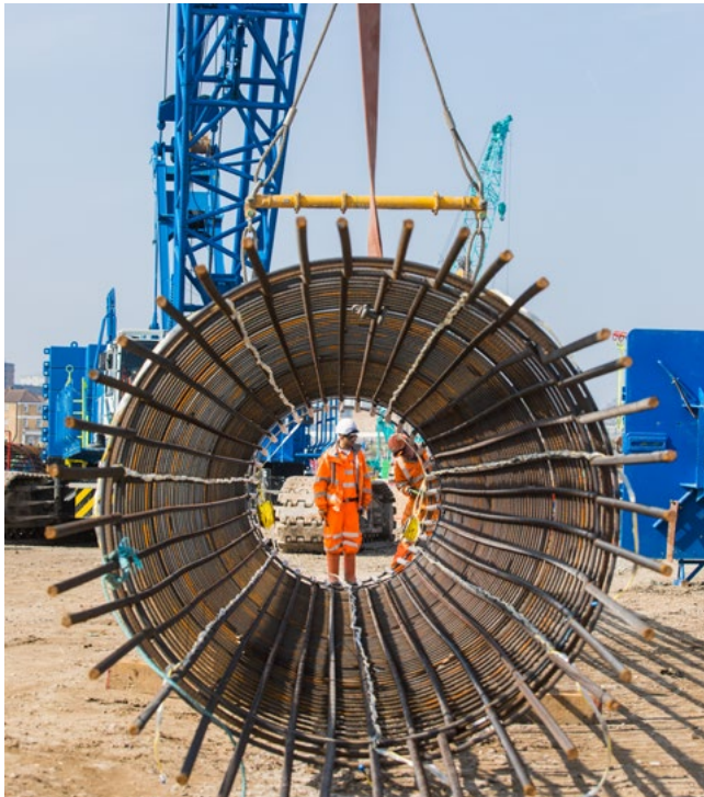
Construction work at Old Oak Common station in west London.
