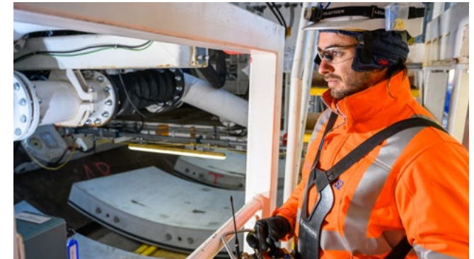
A tunnel boring machine operator at Long Itchington Wood.
