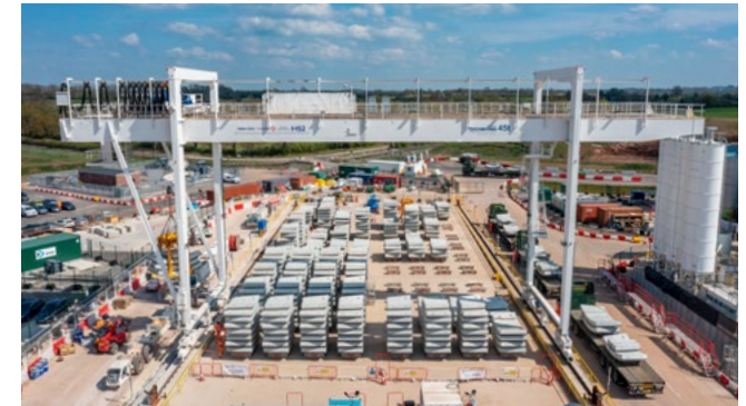
Girder gantry crane at Long Itchington Wood.
