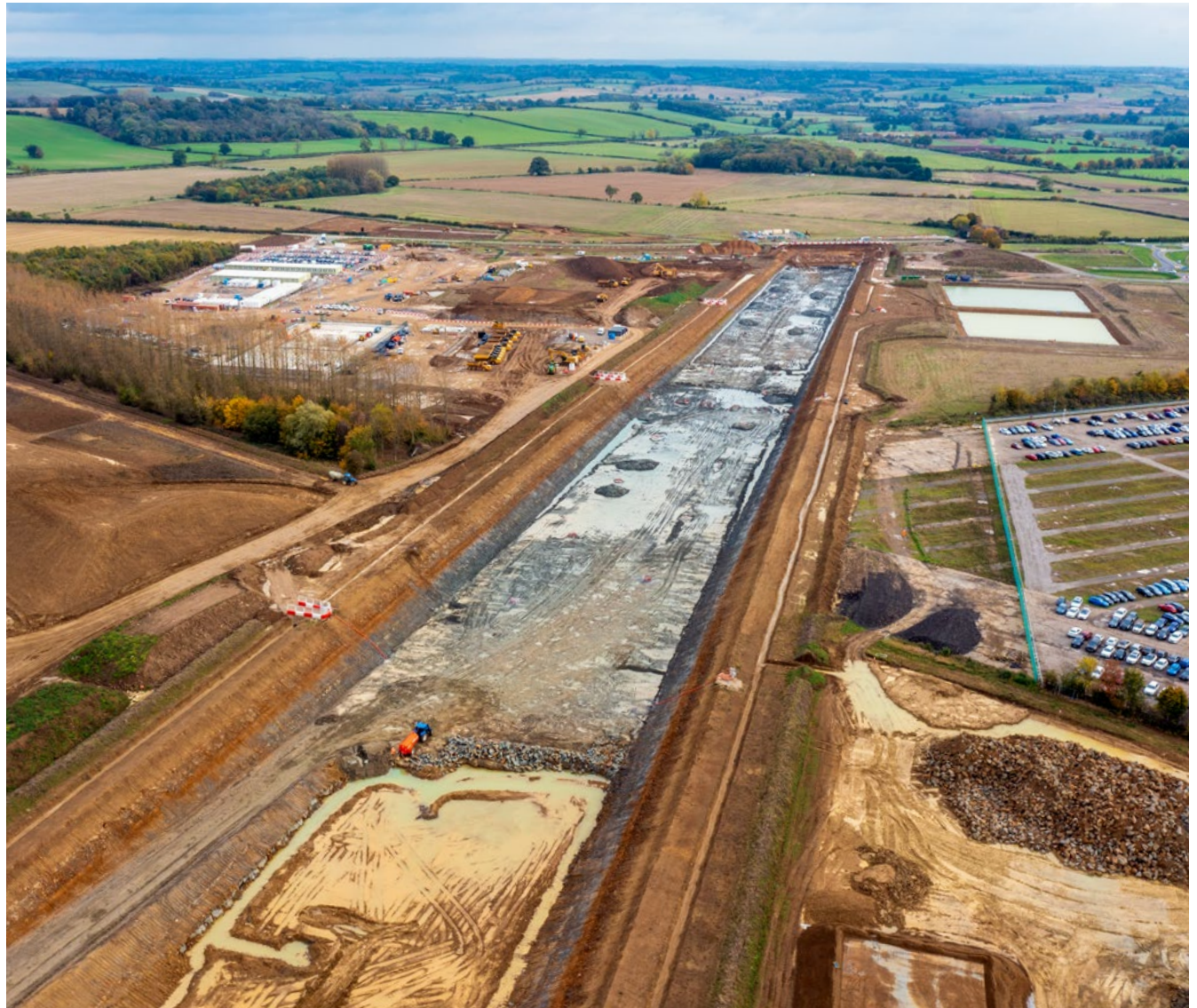
The Chipping Warden 'green' tunnel site in Northamptonshire.
