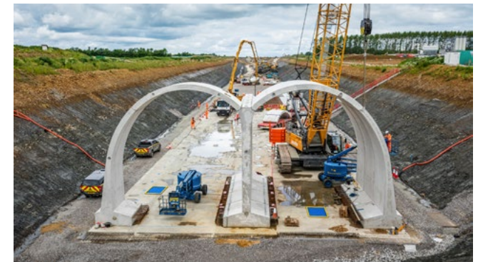
Building the 'green' tunnel in Chipping Warden.
