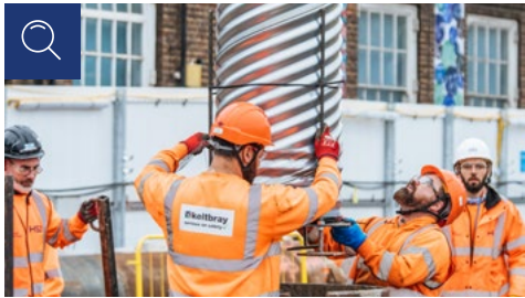
A HIPER pile being installed in central London.
