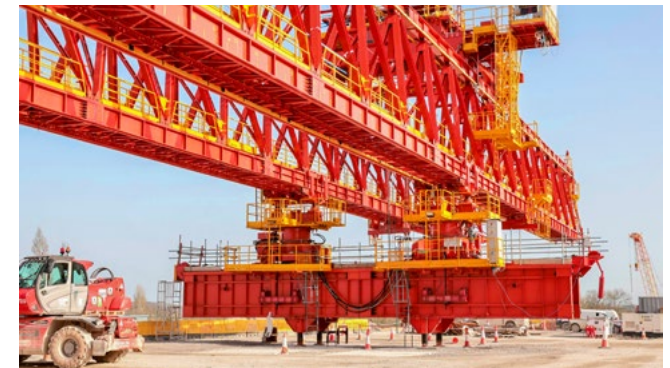
The launching girder for the Colne Valley viaduct.
