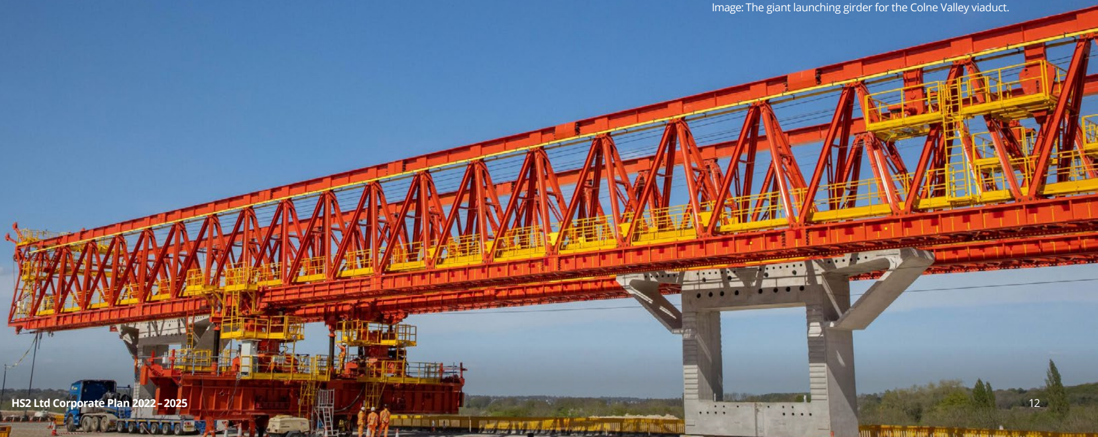
Image: The giant launching girder for the Colne Valley viaduct.
