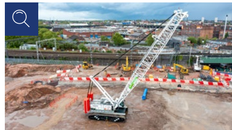
An electric crane at Curzon Street station.
