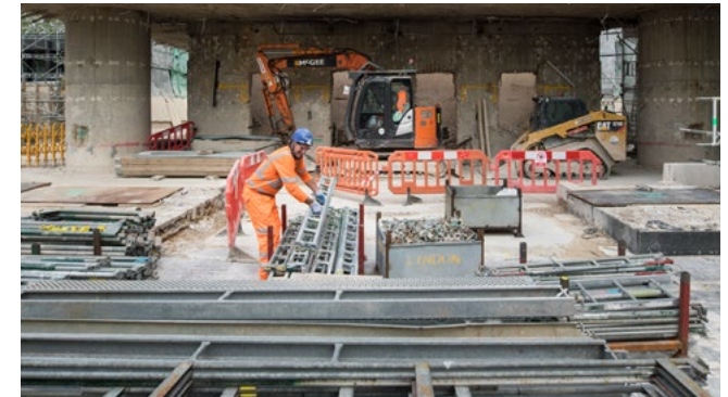
Construction work in progress at Euston.
