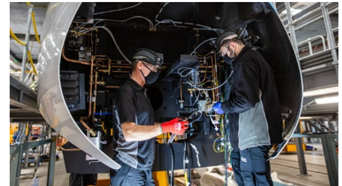
Preparing wiring inside the nose cone of a train at the Hitachi factory where some of the HS2 trains will be manufactured.
