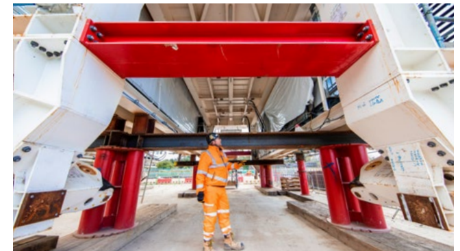
Making checks on a tunnel boring machine.
