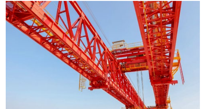
Colne Valley viaduct launching girder.
