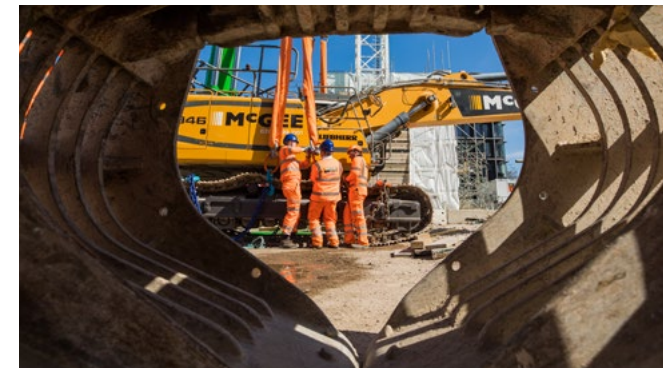
Preparing for a crane lift in Euston.
