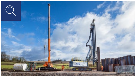
Sheet piling being installed for the Wendover Dean viaduct.
