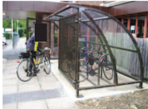
Covered shelter secured with lockable gates
