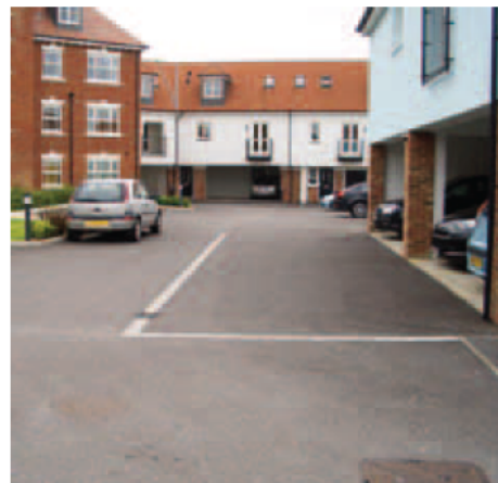
Visible undercroft parking
