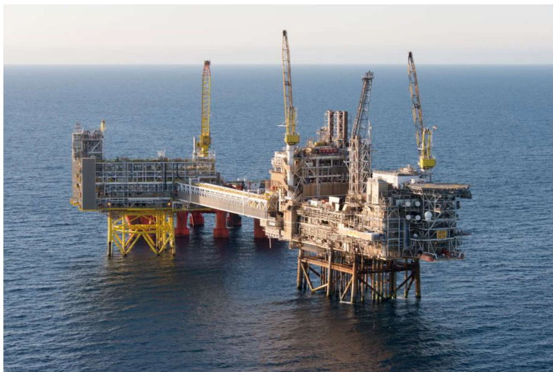
Figure 3-4 Judy Platform complex
