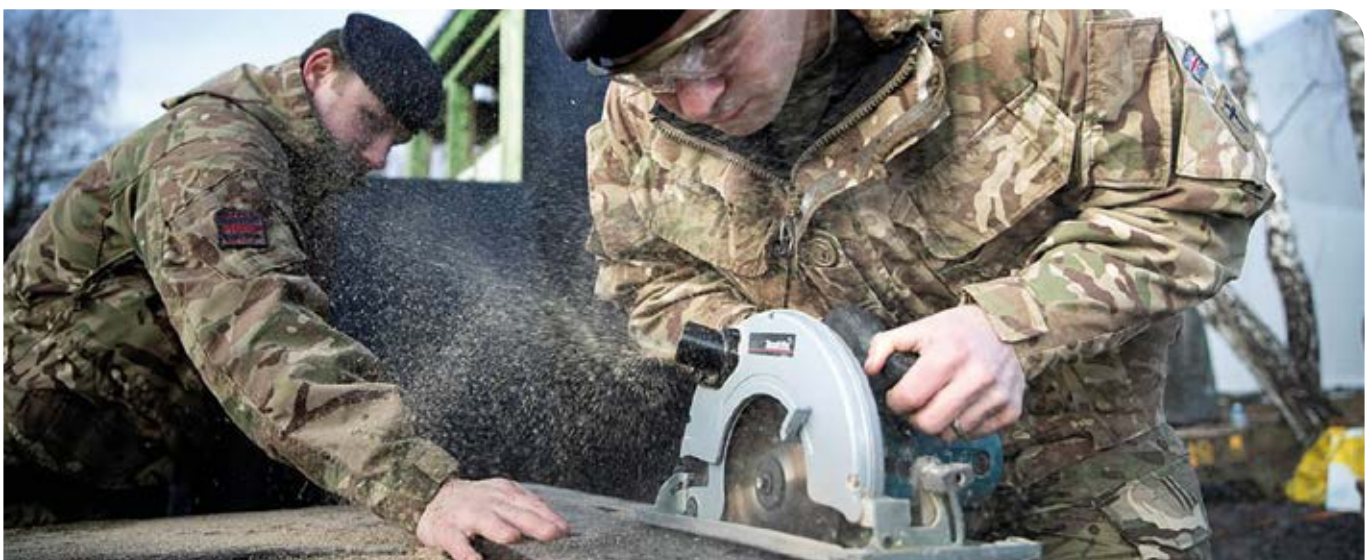
32 Engineers Regiment use specialist carpentry skills to build the first prototype concept Observation Post
