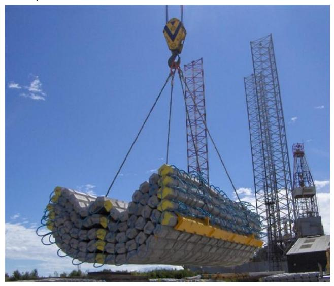
Figure 5.4.2: Speedloader lifting frame<sup>21</sup>
