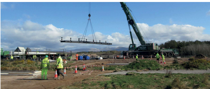
Bridge being installed in sections using huge crane
