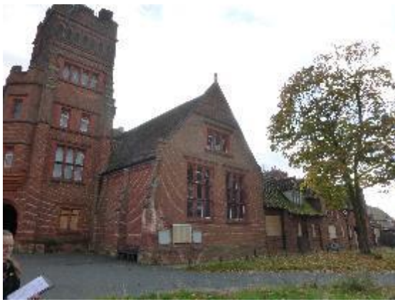
Photo 1. Northern elevation of B1.
