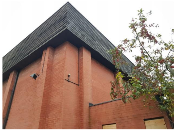
Photo 4. South-western elevation of B21 (Sports Hall).
