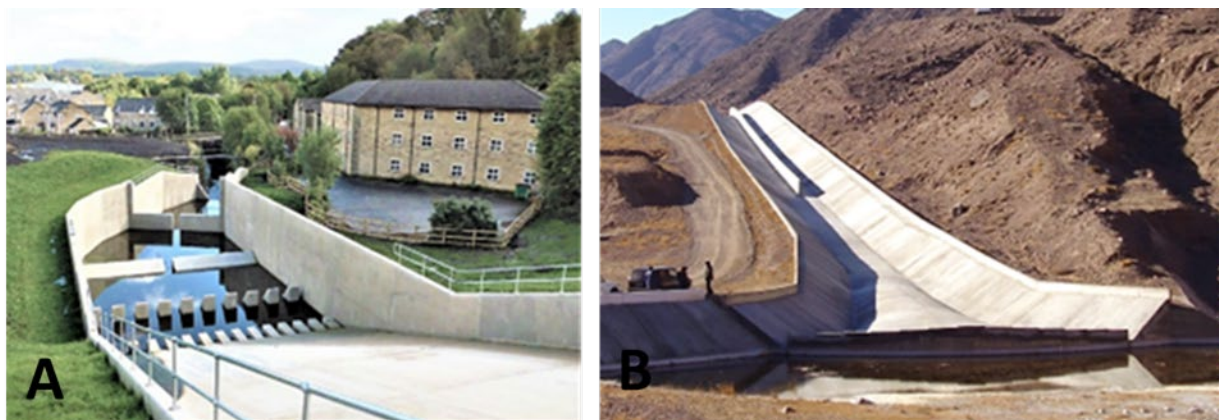
Figure 2.3: Energy dissipations structures. a) USBR type III stilling basin controlled by an end sill at Holdenwood Dam, UK (Source: United Utilities). b) Russian type flip bucket energy dissipator with a splitter wall, double curvature and diverging in plan at Orto Tokoi Dam, Kyrgyzstan (Source: J. Hinks)
