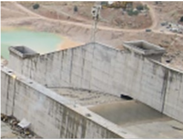
Figure 4.5: Vertical steps and aeration orifices in a smooth reinforced concrete chute at Upper Gotvand, Iran (Source: A. Zia)
