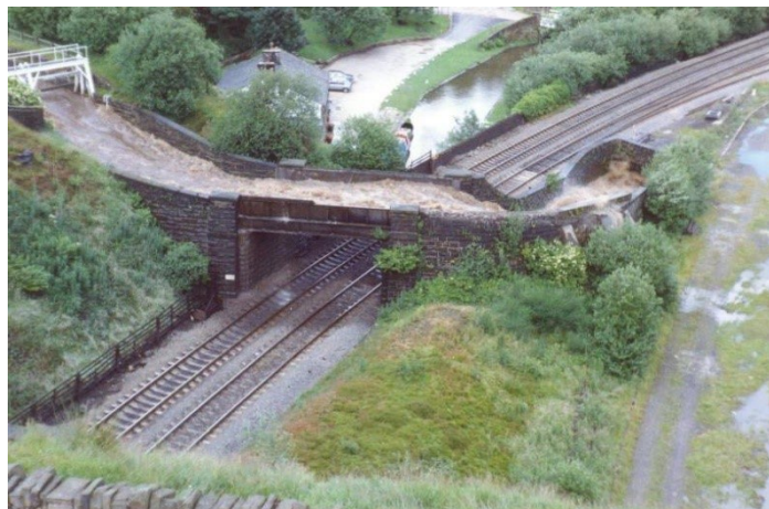
Figure 6.8: Spillway chute with sharp bend built over a railway line and subject to shock waves at the bend (Source: D.Brown)
