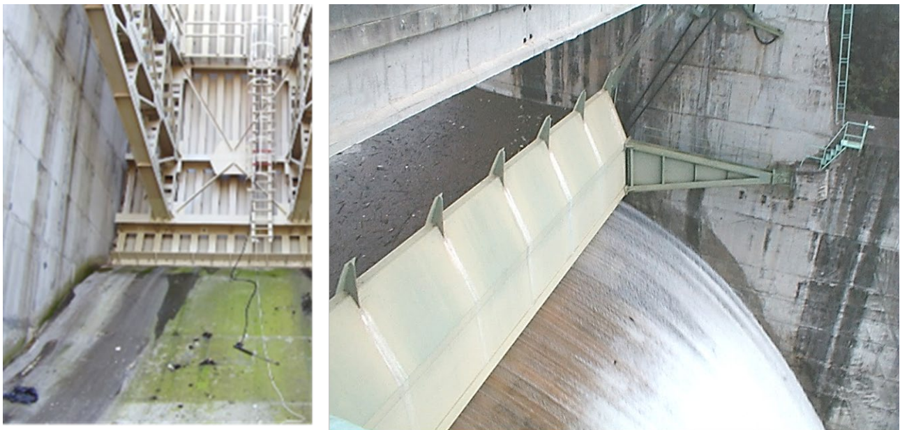
Figure 6.6: Gated overflow structure crest profiles achieving smooth flow conditions without flow separation (Source: J. Hinks)
