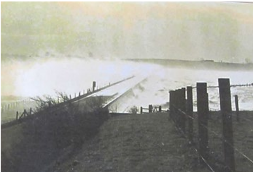
Figure 4.5: Spray due to breaking waves blown over the embankment and downstream shoulder (Source: South Staffordshire Water)
