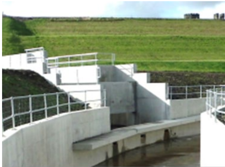
Figure 6.13: 'Impact' type energy dissipator and receiving channel, Ogden Dam, UK (Source: United Utilities)
