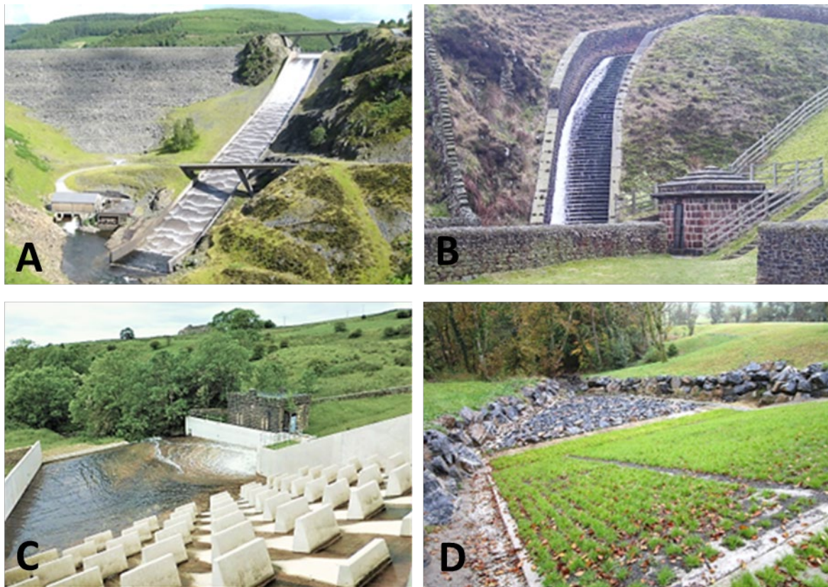
Figure 2.2: Typical conveyance structures (chutes). a) Smooth straight reinforced concrete chute during operation with roll waves, Llyn Brianne Dam, UK (Source: J. Hinks). b) Stepped stone masonry chute, curved in plan, Ogden Upper Dam, UK (Source: United Utilities). c) Baffled chute and stilling basin, Lee Green Dam, UK (Source: V. Pavlov). d) Cable-tied reinforced grass auxiliary spillway, Llyn Mawr Dam, National Botanic Garden of Wales, UK (Source: J. Hinks)
