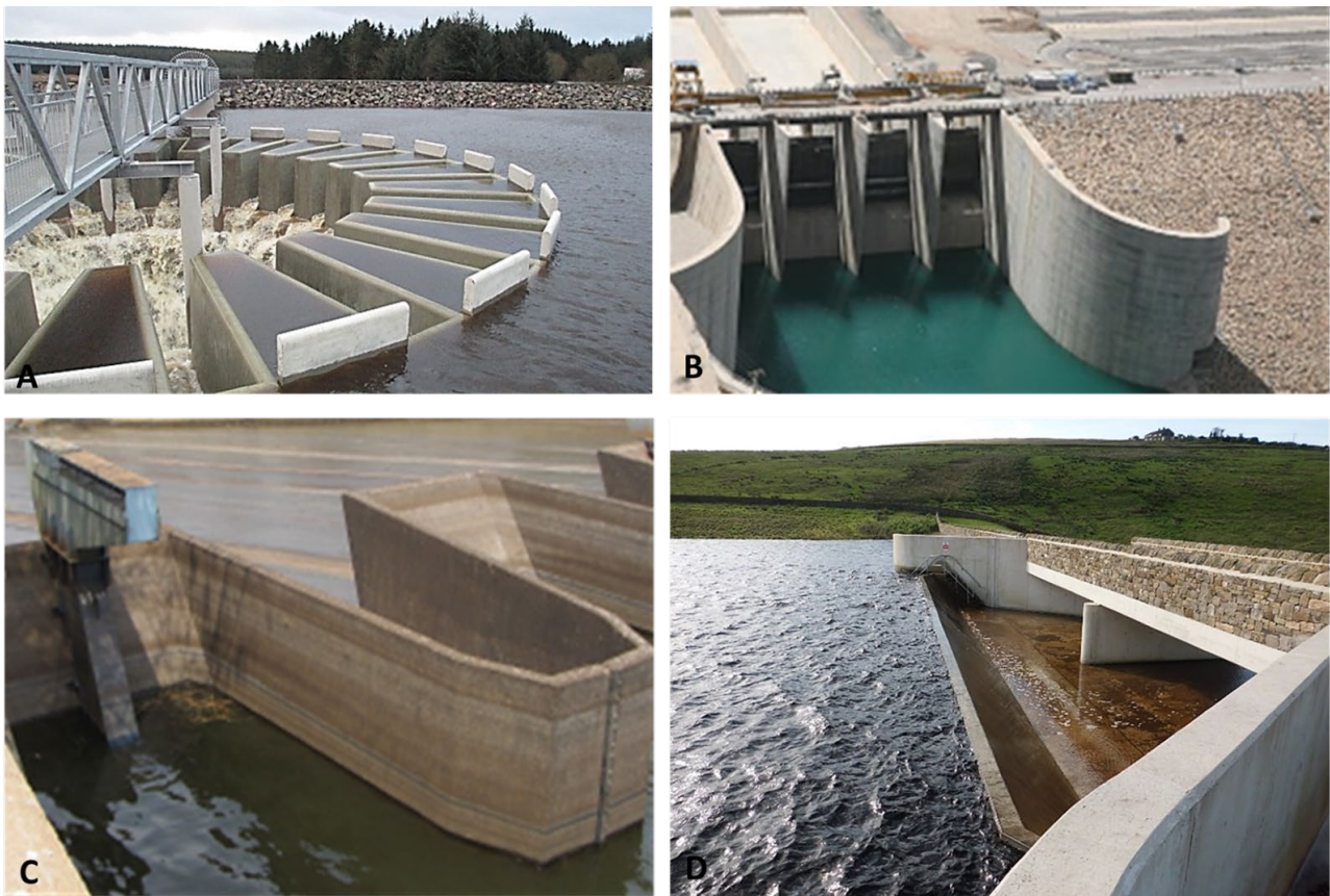
Figure 2.1: Inlet structure arrangements. a) Piano-key weir with submerged inlet baffles providing control of floating debris, Black Esk Reservoir, UK (Source: J. Ackers). b) Gated weir equipped with radial (segment) gates, Upper Gotvand Dam, Iran (Source: A. Zia). c) Tipping gates forming a labyrinth weir, Kamuzu Dam II, Malawi (Source: J. Hinks). d) Trapezoidal inlet weir followed by a converging transition to the downstream conveyance structure, New Year’s Bridge Dam, UK (Source: V. Pavlov)
