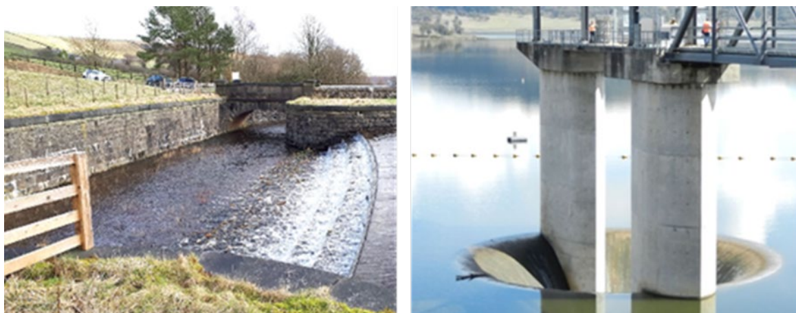
Figure 6.4: Curved crest overflows with large radius (left) and small radius (right) (Sources: V Pavlov (left) and Binnies UK Ltd. (right))
