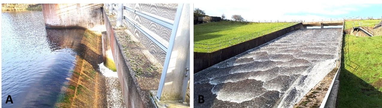
Figure 6.1: Straight overflow structure followed by a conveyance structure of the same width designed for high unit discharge, Holdenwood Dam, UK (Source: V. Pavlov)
