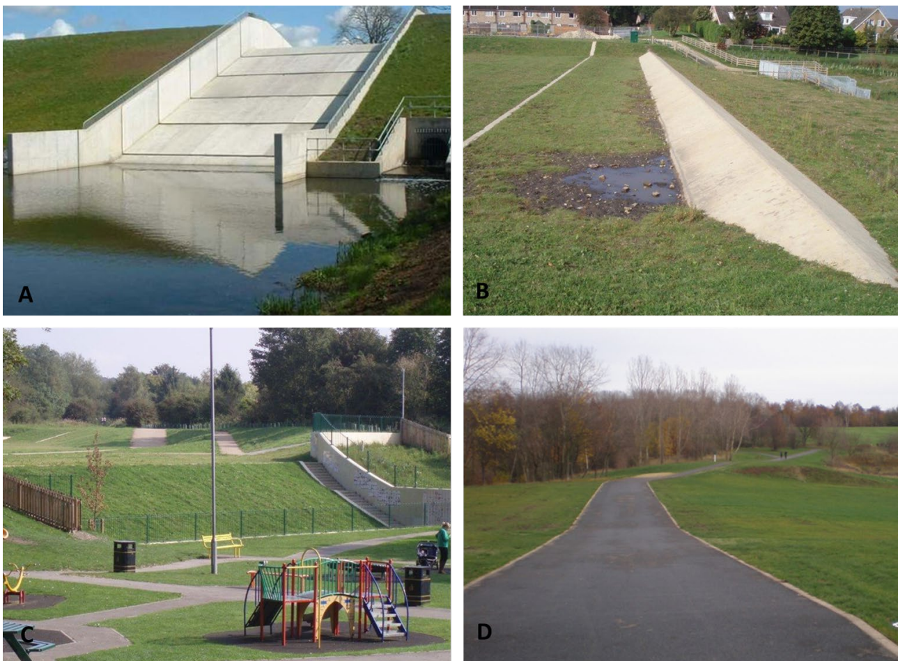
Figure 11.1 Risk to public safety posed by spillway structures (Source: Glen Brady). a) Undrained stilling basin and its wing walls used as diving points. b) Exposed spillway structure with steep slopes within a heavily used public area. c) Spillway flow route passing through a children's playground and well used park area. d) Public pathway used a spillway crest structure
