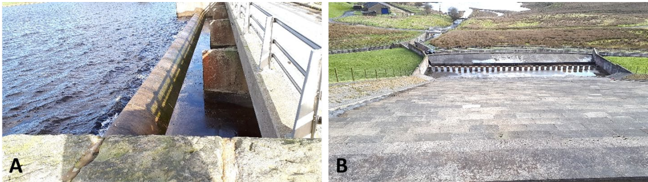
Figure 6.2: Straight overflow structure followed by a low-cost or flexible conveyance structure designed for low unit discharge, Ogden Dam, UK (Source: V. Pavlov)
