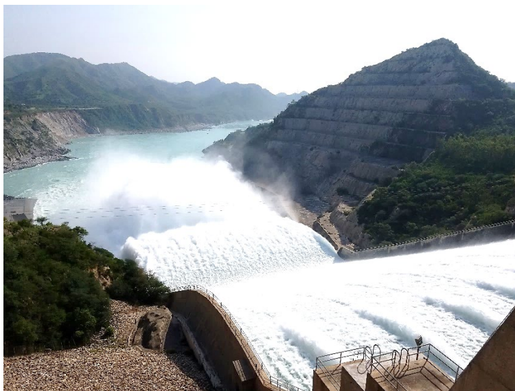
Figure 6.14: Ski-jump energy and plunge pool energy dissipator under operation with highly aerated flow, Tarbela Dam, Pakistan (Source: J. Hinks)
