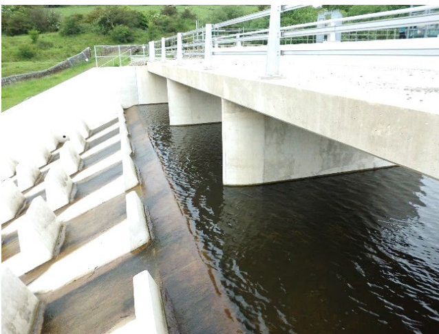
Figure 6.10: Baffled apron chute and inlet structure with crest bridge, Lee Green, UK (Source: V. Pavlov)
