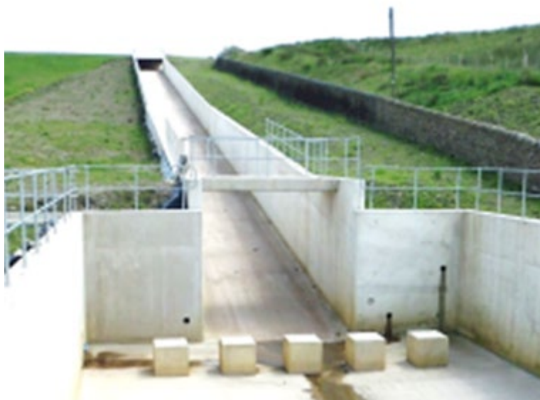
Figure 6.12 Spatial hydraulic jump stilling basin with baffle blocks at the inlet to the basin. Swinden I Dam, UK (Source: V. Pavlov)
