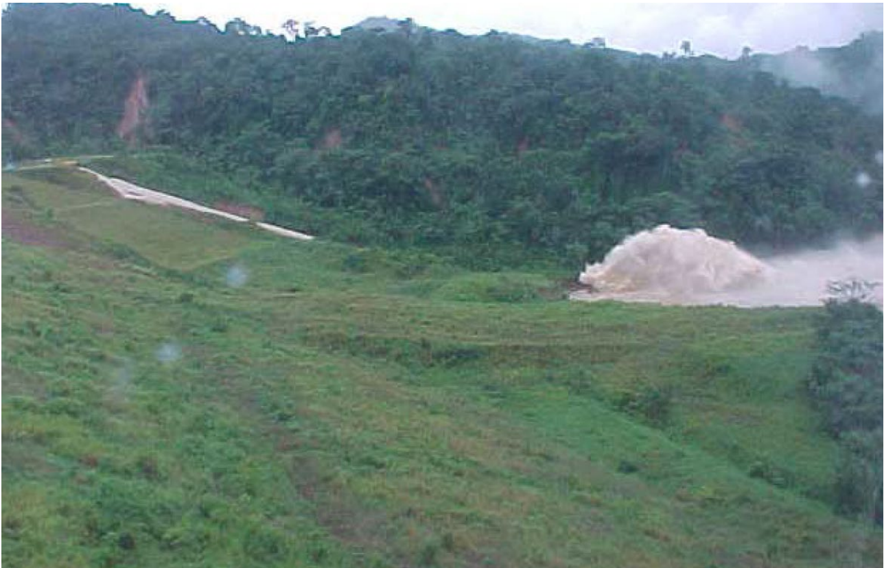
Figure 4.4: Stilling basin sweepout resulting from insufficient tailwater depth or stilling basin length (Source: USBR)
