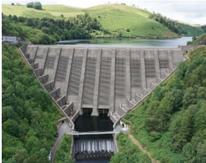
Figure 6.9: Modern concrete stepped spillway on the face of a concrete gravity dam discharging onto large stepped reinforced concrete channels built on the abutments, Clywedog Dam, UK (Source: N. Prytherch)
