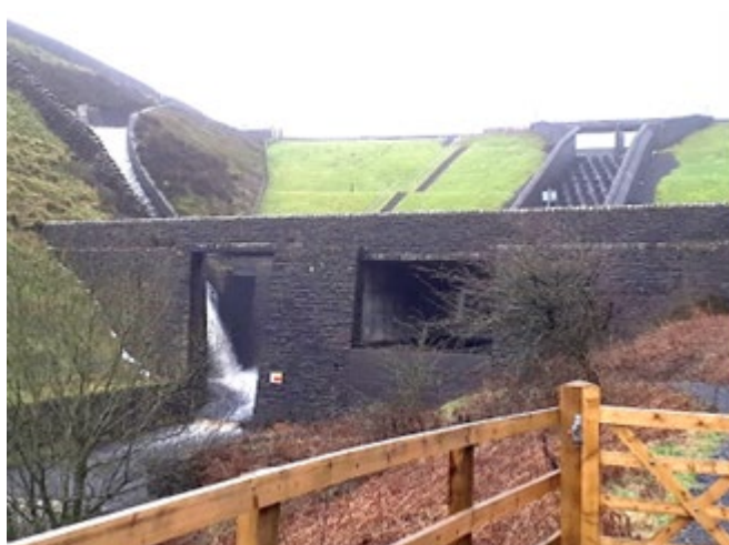
Figure 4.1: Ogden Upper Reservoir. Main stone masonry spillway on the abutment and auxiliary baffle spillway on the embankment (Source: V. Pavlov)
