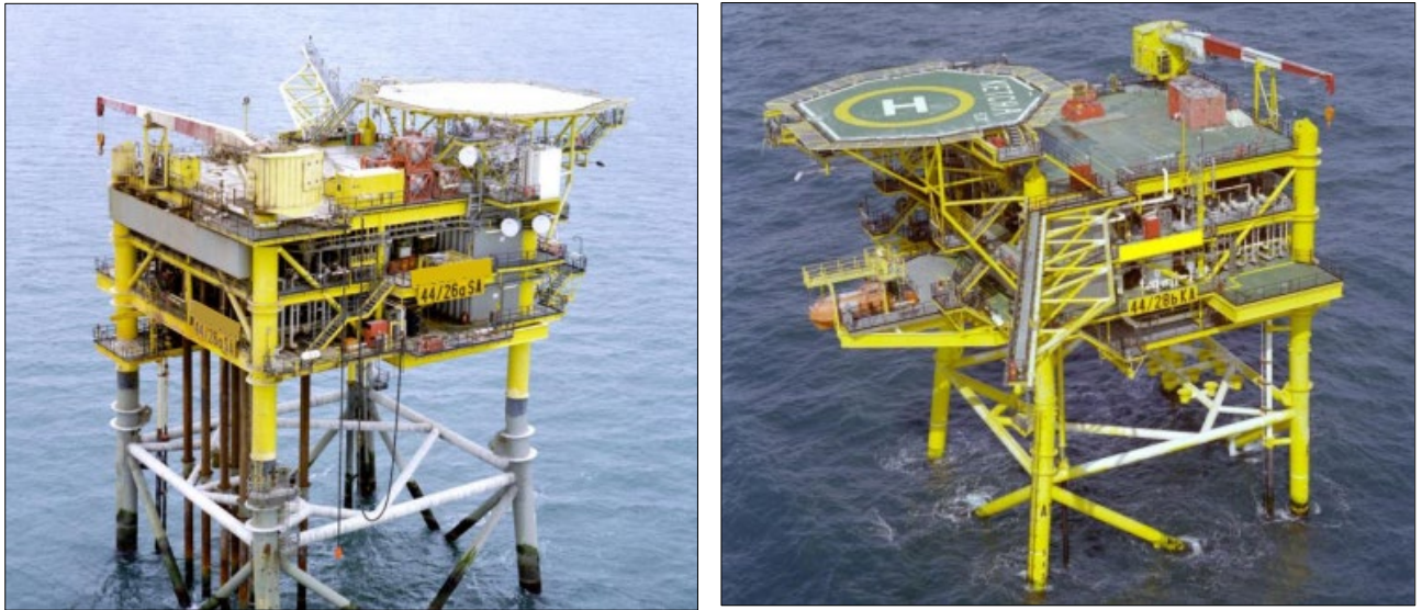
Figure 2: Schooner and Ketch Normally Unmanned Installations (NUIs).
