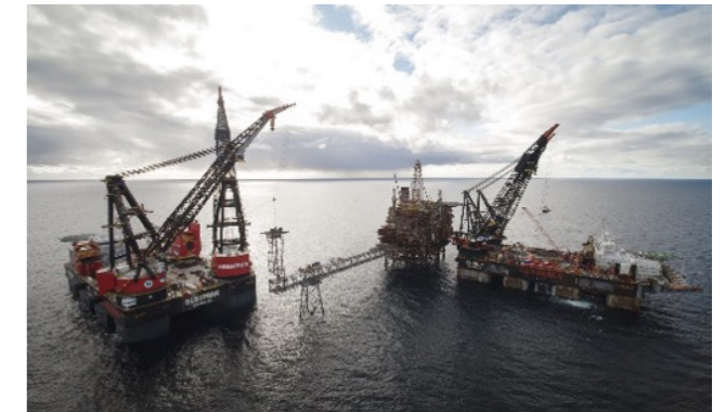
Brae Bravo topsides removal
