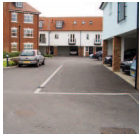
Visible undercroft parking
