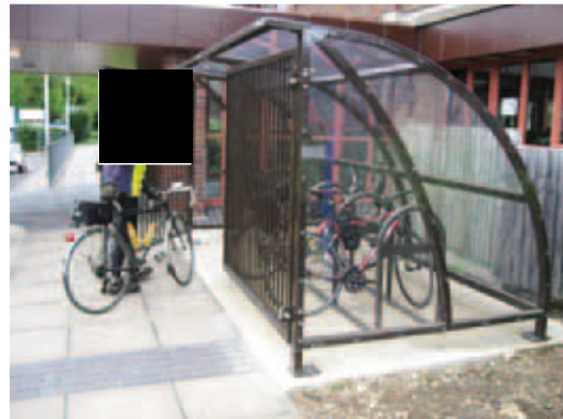
Covered shelter secured with lockable gates
