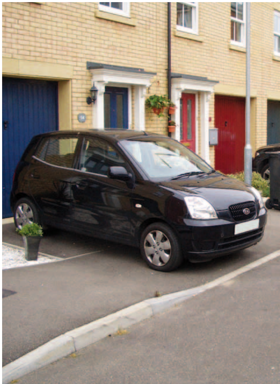
Setbacks from garages and gates lead to vehicles parking in front of garages and blocking footways
