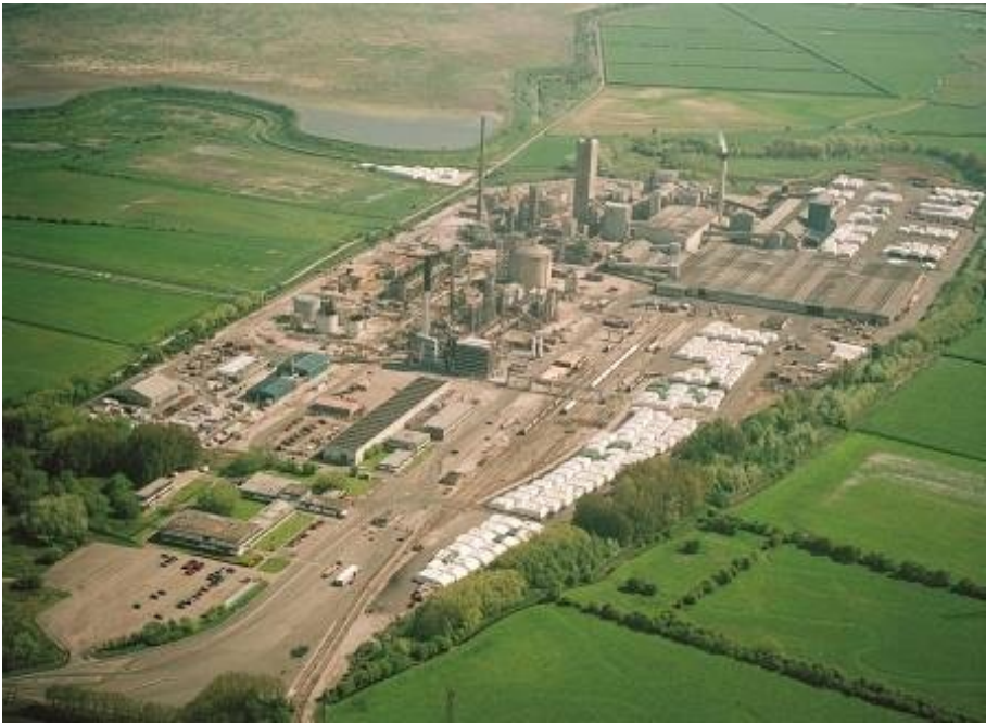
Figure 2.2: View of CF Fertiliser Plant
