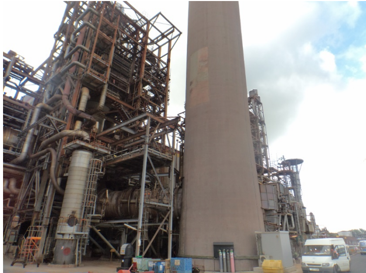
Figure 9.2 Lower Stack Access Point
