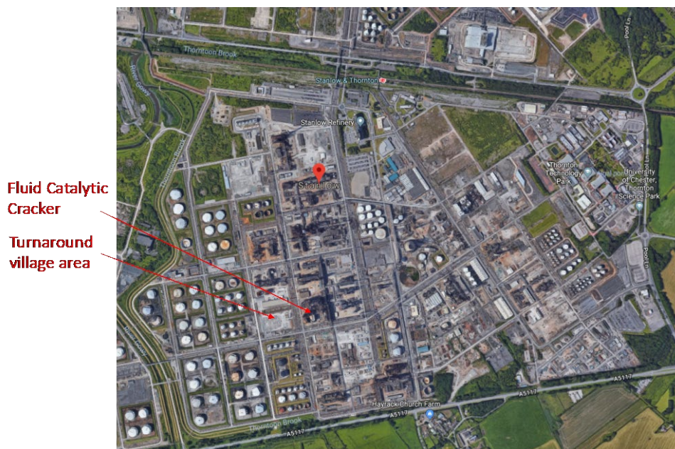
Figure 21 - Stanlow Site showing location of Catalytic Cracker Unit (CCU)
