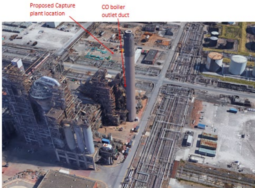
Figure 22 - Stanlow Catalytic Cracker Unit (CCU) illustrating plot constraints
