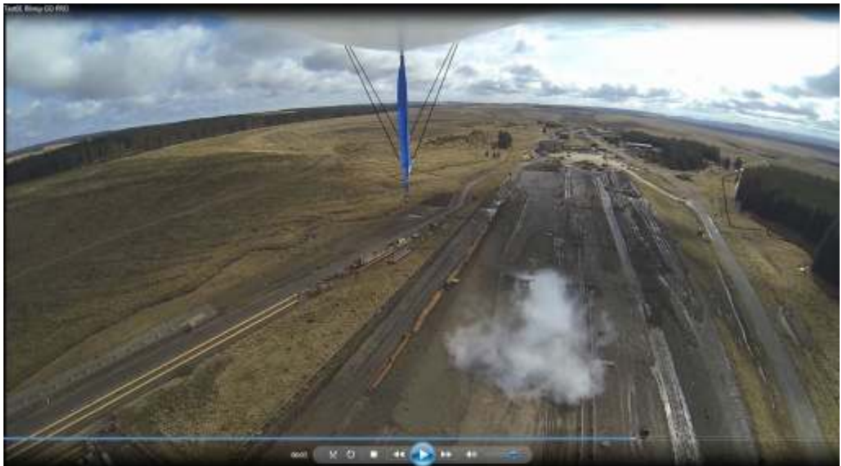
Figure 31(n): Aerial View at Time 360 s from Rupture
