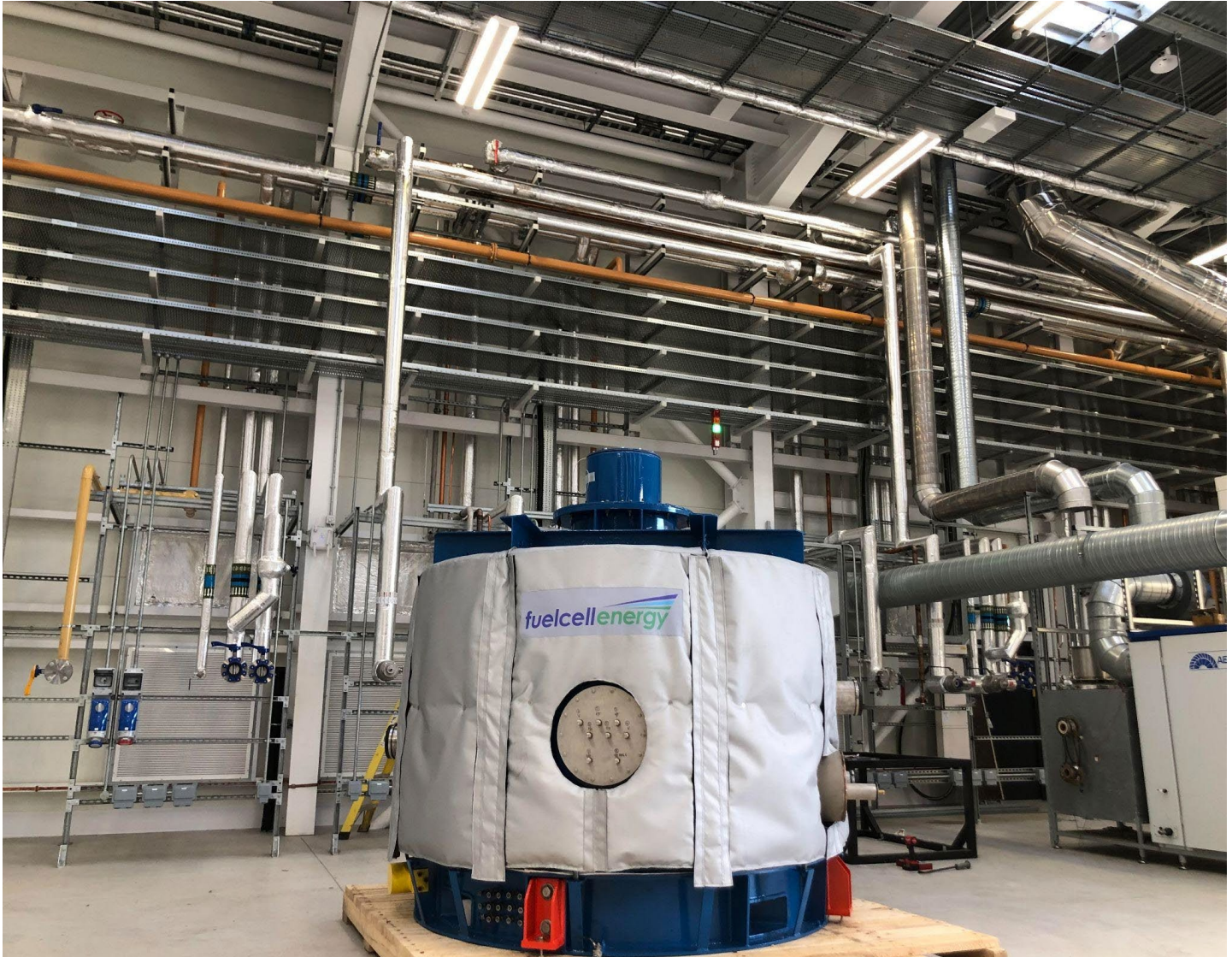
Figure 3: MCFC Installation
