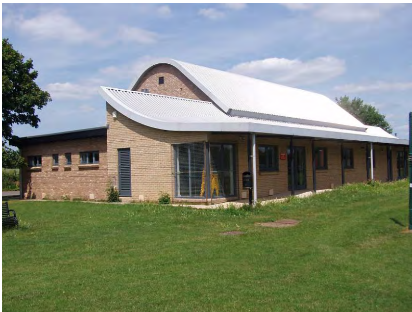
A 'High quality' facility at Great Chesterford Community Centre
