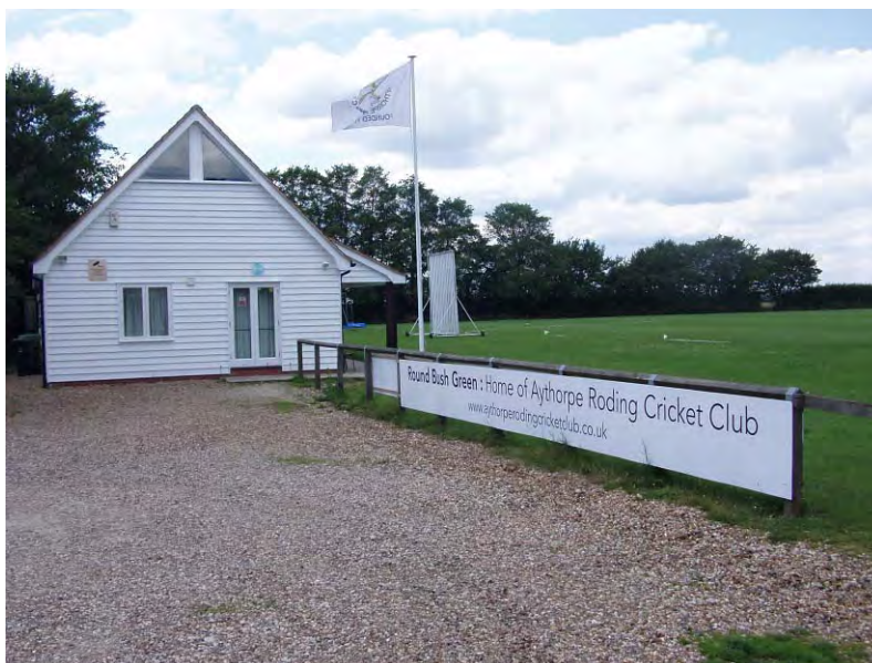
A good quality pavilion serving football and cricket at Roundbush Green
