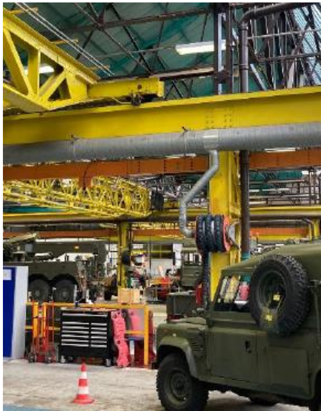
Photograph 2: Fan motor assembly and motor was found on the workshop floor where the cone is placed.
